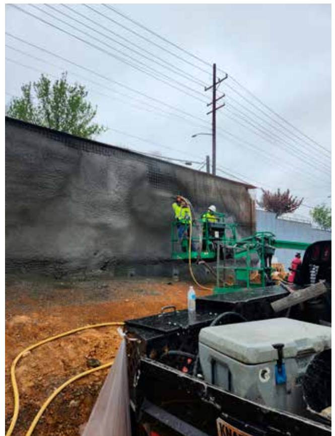
Fig. 3: Crews shotcreted over a reinforced soil nail wall facing during construction.
