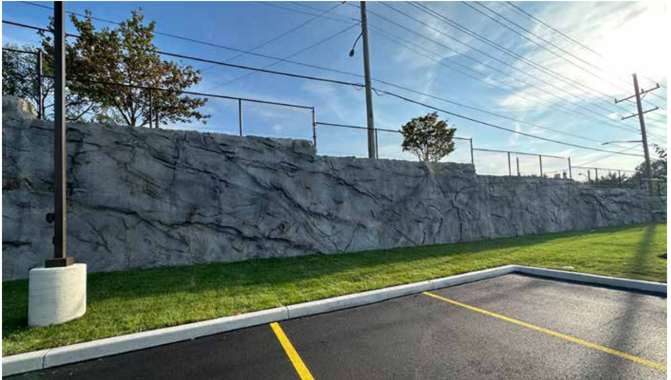
Fig. 1: The completed, sculpted, and stained shotcrete wall provides permanent support for the roadway above while creating an architectural finish for the redeveloped site. The finished retaining wall combines soil nail stabilization with sculpted concrete facing, preserving usable site area while supporting Northern Avenue above.
