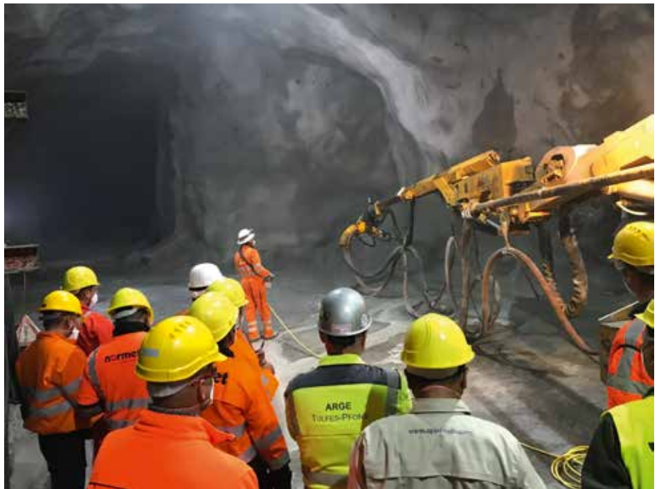
Fig. 1: Shotcreter education in full swing
