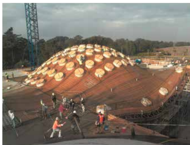
Fig. 1: The 'rolling roof' of California Academy of Sciences in San Francisco, in progress.
