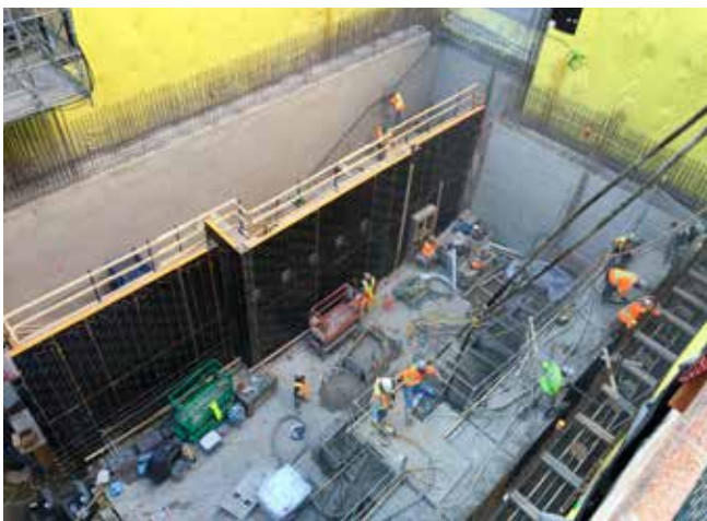
Fig. 1: Mount Pleasant LRT station on Toronto's Eglinton Crosstown line. The 2022 ASA Infrastructure Project of the Year Award-Winner incorporated UltraFiber 500 micro-cellulose fibers in the 70% slag shotcrete mixture for its 1.5 m (4.9 ft) thick, heavily reinforced underground walls. All photos courtesy of Shaun Radomski, M.Sc., P.Eng. Senior Materials Engineer Thurber Engineering Ltd.
