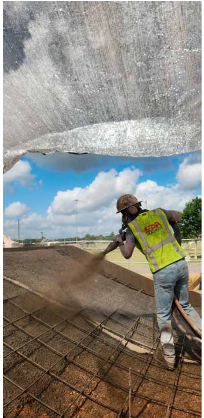
Fig. 6: Providing shade to the area being shotcreted provides immense benefits while shooting in the heat
