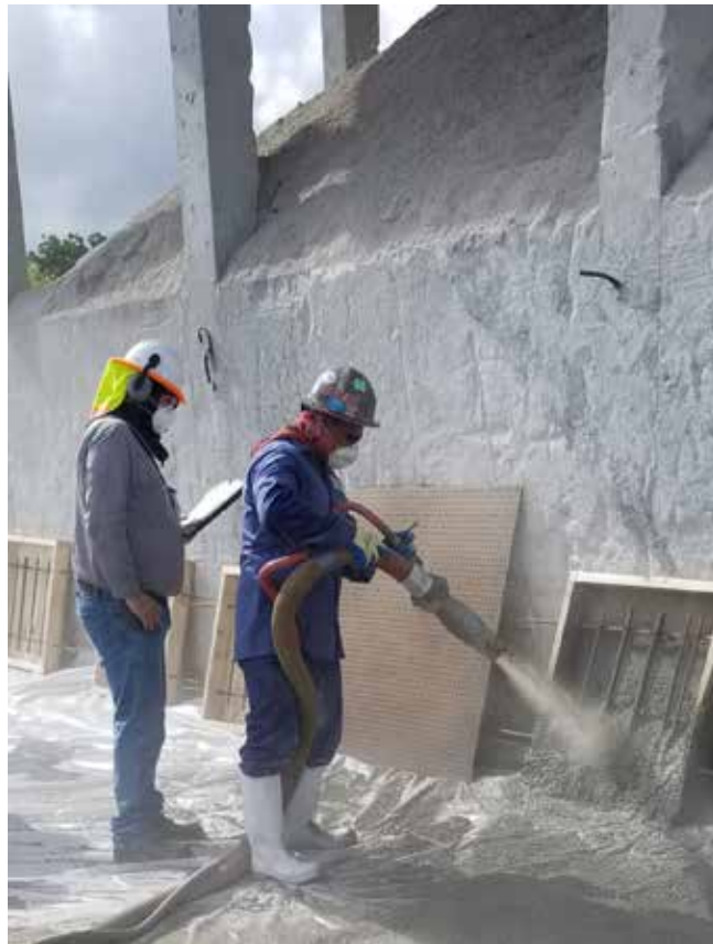
ACI Shotcrete Inspectors help ensure quality shotcrete placement
