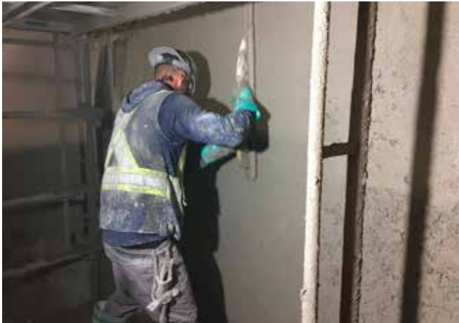
Fig. 3: Wooden floats were used to close the surface.
