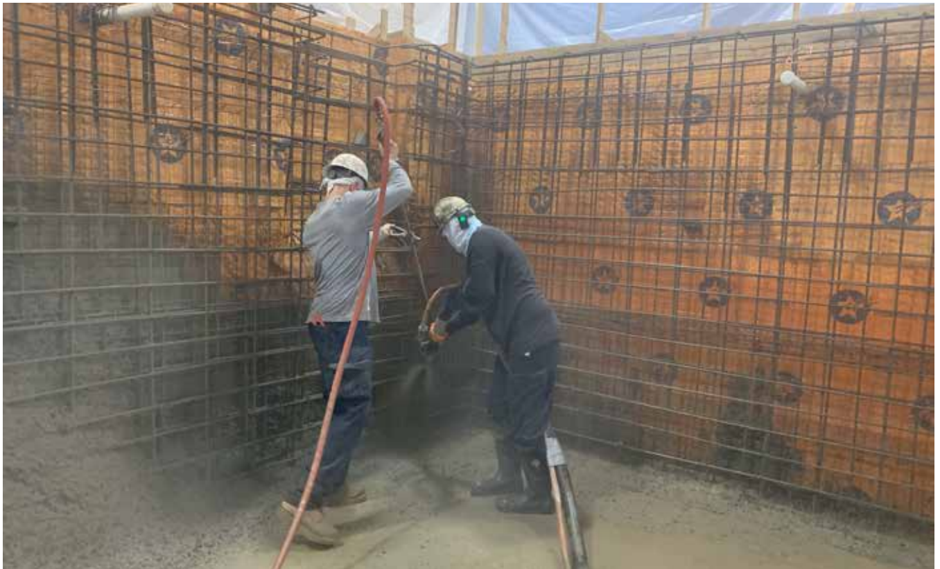
Fig. 5: ACI-certified shotcreter Mason Guarino working with a blow pipe operator to ensure a monolithic floor-wall joint is shotcreted
