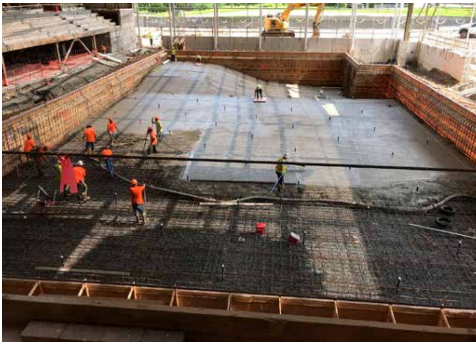
Fig. 1: Large pool floor being placed with a line pump system and 4 in. (100 mm) concrete line on an indoor pool
