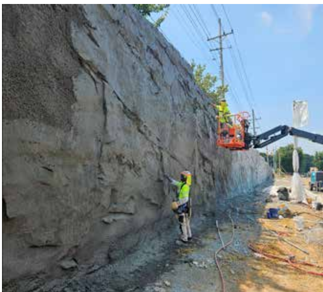
Fig. 2: Crew members sculpt the shotcreted facing to create a natural rock appearance integrated into the retaining wall system.
