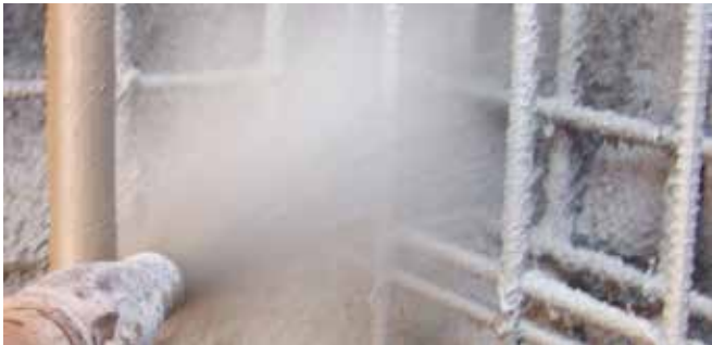
Fig. 2: High velocity shotcrete placement in a wall
