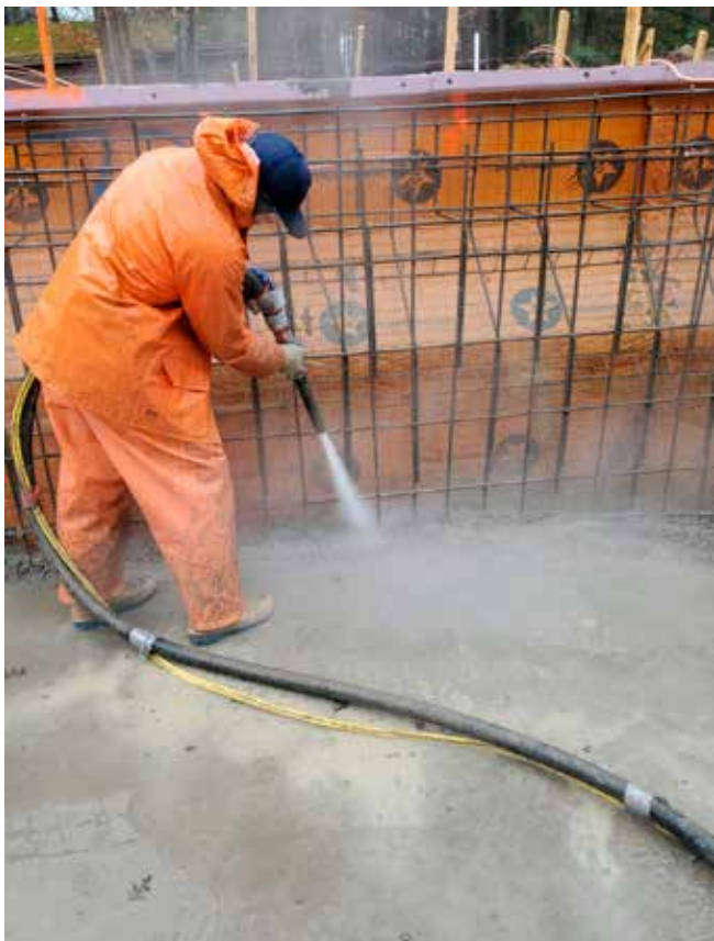
Fig. 4: Slurry blasting to clean a future wall joint location
