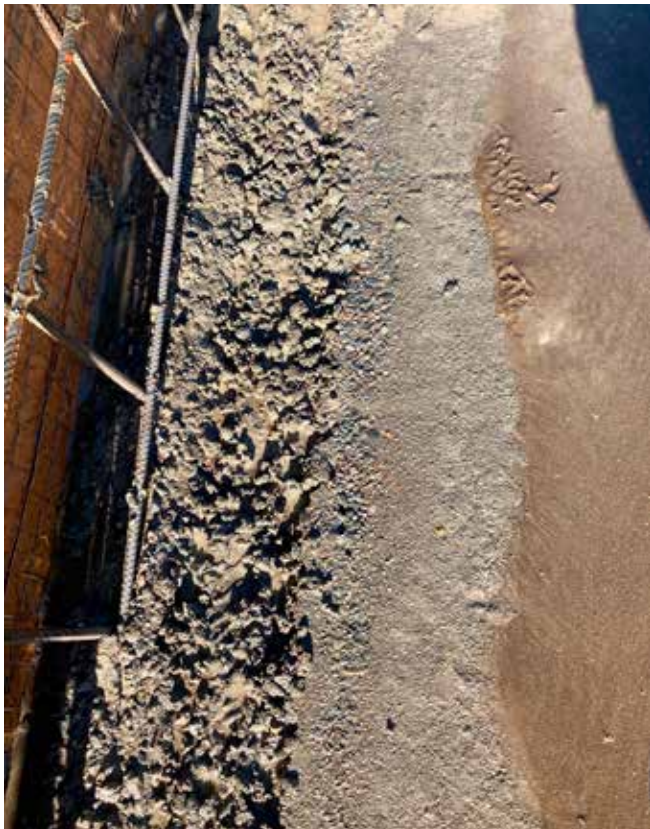
Fig. 3: Roughened finish at the floor-wall joint to receive shotcrete
