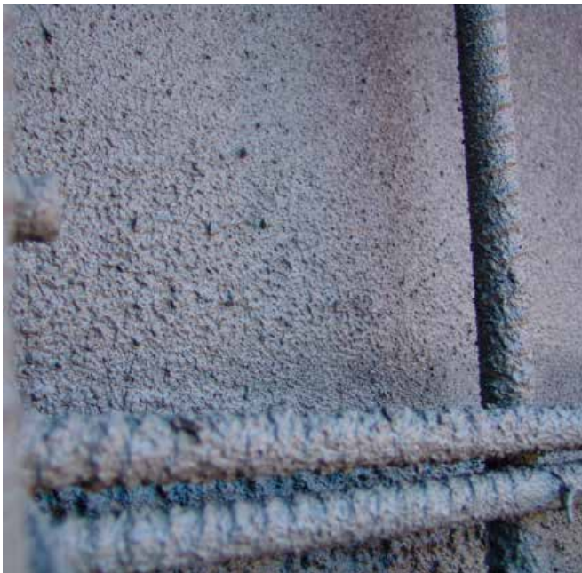
Fig. 3: Initial paste-rich shotcrete placement without coarse aggregate
