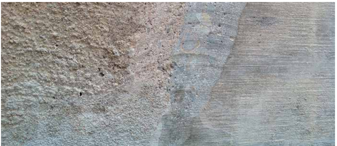
Fig. 6: Intimate contact and full bond of new shotcrete placement (right, gray) with old concrete (left, beige)
