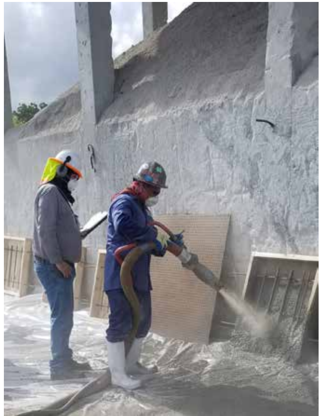
ACI Shotcrete Inspectors help ensure quality shotcrete placement
