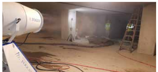
Fig. 7: Utilizing a fog cannon to provide moisture in the air during hot weather shotcrete
