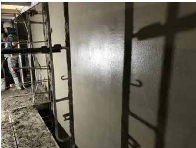
Fig. 4: In this close-up review of the steel trowel finish wall, the shotcrete mix incorporates 70% slag cement and UltraFiber 500, displaying excellent finishability, creating finished surfaces without any pulls or tears.
