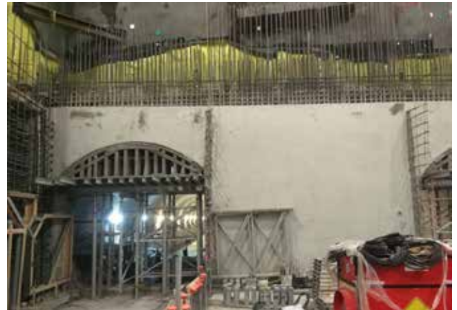
Fig. 5: The finished surfaces were free of voids, sags, tears, or plastic shrinkage cracks attributed to the use of the UltraFiber 500 Cellulose Micro-Fiber.
