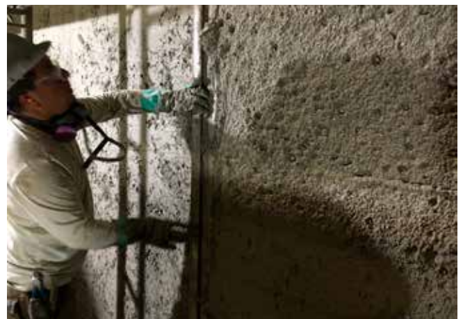
Fig. 2: Final coat was shot, cut, and finished to the specified line and grade of shooting wires. UltraFiber 500 alkali-resistant cellulose fiber was incorporated into the mixture to enhance pumpability, shootability, adhesion, cohesion, stackability, and finishability of the mixture.
