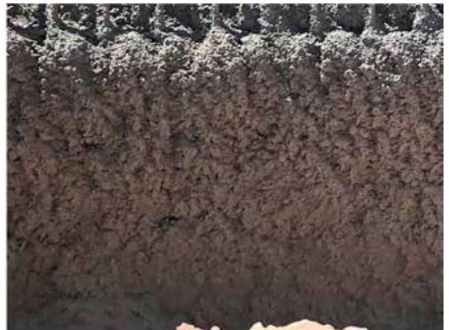
Fig. 8: Wrong angle shooting results in surface waviness
