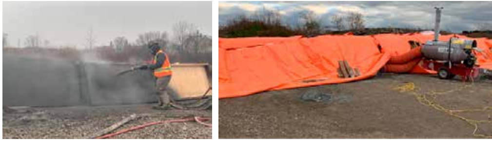
Spraying the panels and outdoor curing
