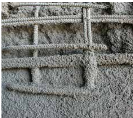
Fig. 6: Sandy or dull, opaque surface during placement
