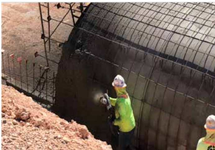
Fig. 8: Wrong angle shooting results in surface waviness
