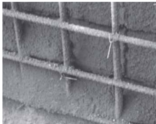
Fig. 6: Sandy or dull, opaque surface during placement
