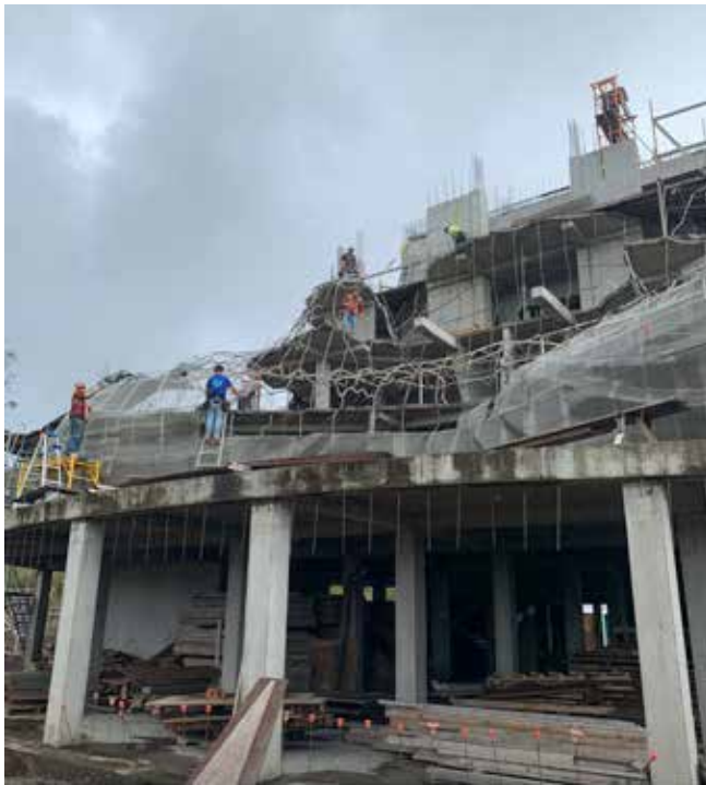
Fig. 3: Adding mesh to armature
