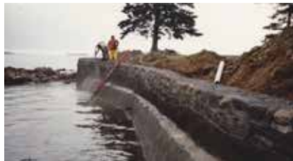
Fig. 4: While working with the 8 ft (2.4 m) tides at various levels the shotcrete placement begins from bottom to top and over the wall down the backside to the newly installed filter fabric and crushed stone backside drainage feature to capture and safely remove the overwash drainage from extreme tides
