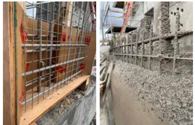
Fig. 4 (ABOVE and BELOW): Preconstruction mock-ups with dry-mix shotcrete for the encapsulation of reinforcement and Sika® Galvashield® galvanic anodes. Photo credit: Sika Canada (2023).
