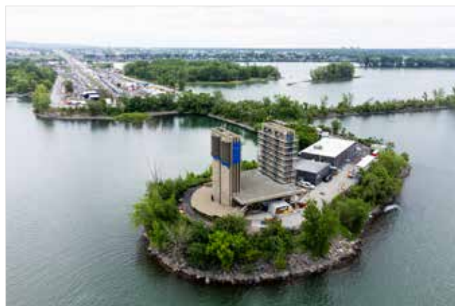
Fig. 2: Ventilation towers of the Louis-Hippolyte-La Fontaine tunnel. Photo credit: La Presse (2024).
