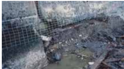
Fig. 3: The same procedure as in #1 was all in preparation of the dry-mix shotcrete placement at various thickness to provide a reasonable looking non troweled finish
