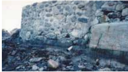
Fig. 1: Cleaning the bottom of the seawall at low tide by fresh water blasting and securing a new "through drains" and placement of new galvanized 2 x 2 WWF, tied to epoxy set 6 in. galvanized anchor bolts on a 2 ft x 2 ft pattern
