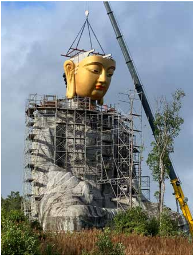
Fig. 7: Lifting parts of the head
