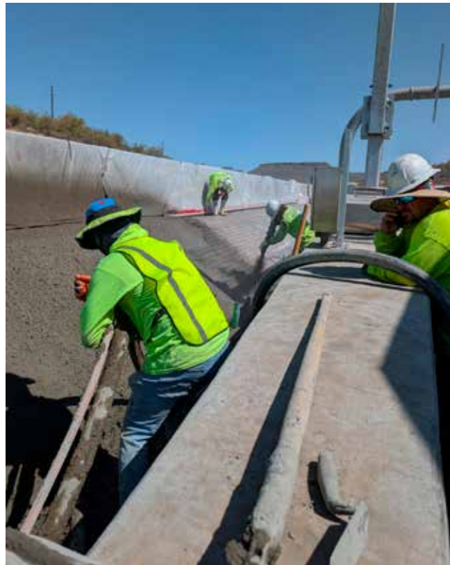
Fig. 3: Shotcrete crew placing concrete on reinforced slope protection along a highway embankment in Arizona
