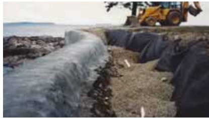
Fig. 2: The final stages of completing the backside drain system up to the top of the seawall
