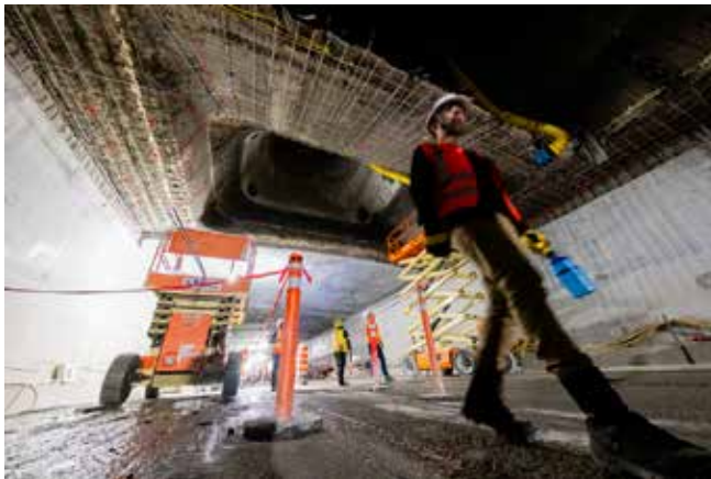
Fig. 3 (ABOVE and BELOW): Views of one of the severely damaged shafts undergoing repair inside the tunnel. Photo credits: La Presse (2024) and Sika Canada (2024).
