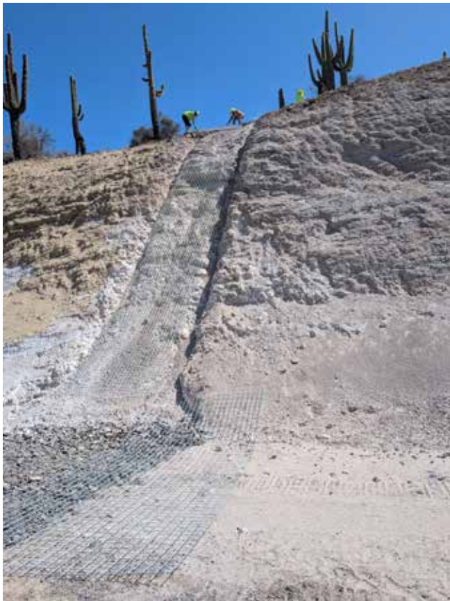
Fig. 2: Rebar installation on a steep slope for the upcoming shotcrete application and erosion control system
