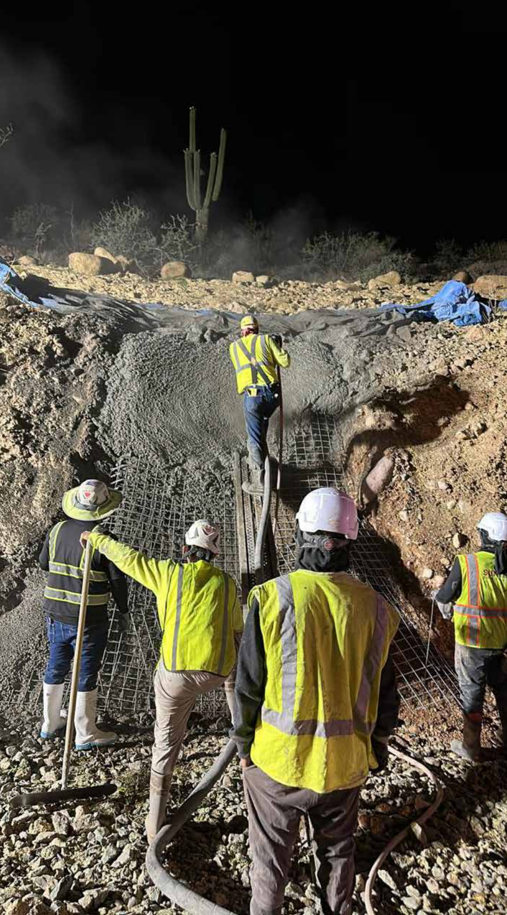
Fig. 4: Shotcrete crew applying concrete over rebar for wash lining and slope stabilization in desert terrain
