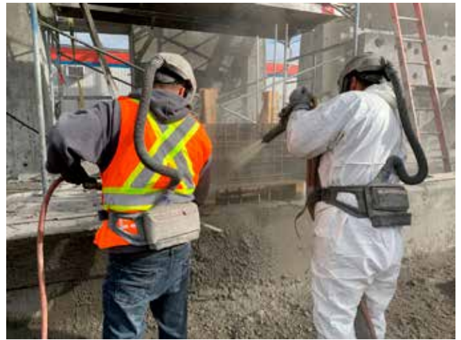
Fig. 4 (ABOVE and BELOW): Preconstruction mock-ups with dry-mix shotcrete for the encapsulation of reinforcement and Sika® Galvashield® galvanic anodes. Photo credit: Sika Canada (2023).
