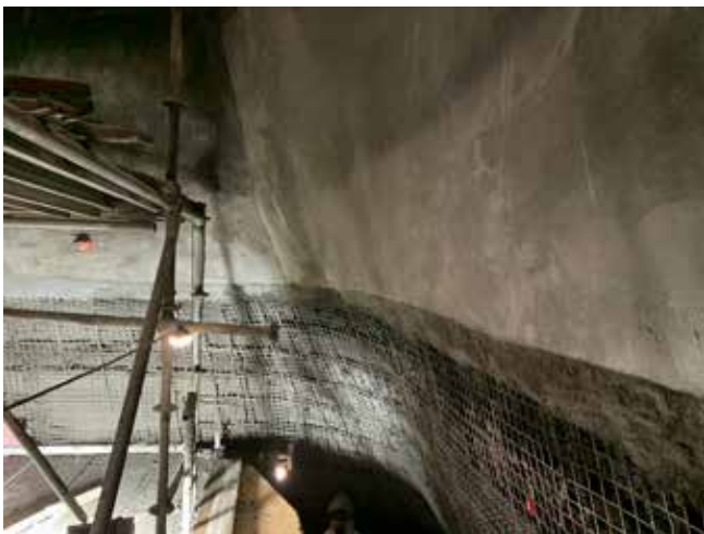
Fig. 3 (ABOVE and BELOW): Views of one of the severely damaged shafts undergoing repair inside the tunnel. Photo credits: La Presse (2024) and Sika Canada (2024).
