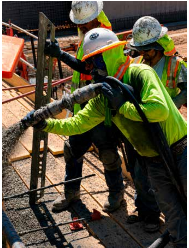
Fig. 3: A shotcreter using proper form for shotcrete placement
