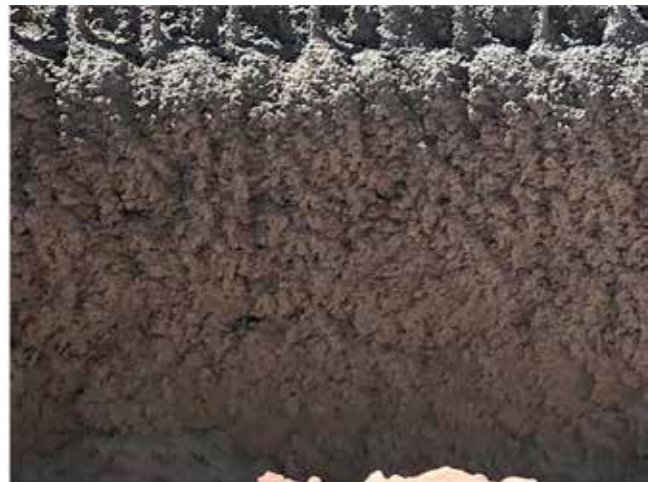
Fig. 8: Wrong angle shooting results in surface waviness
