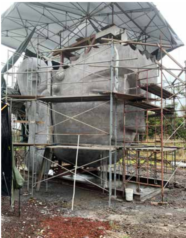
Fig. 2: Head on steel frame
