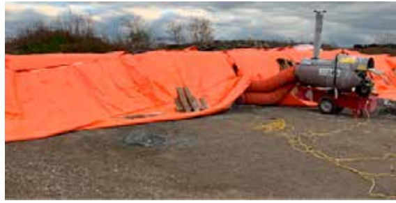
Spraying the panels and outdoor curing
