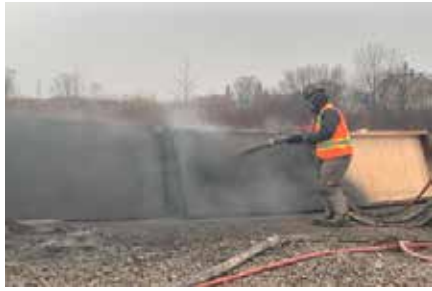
Spraying the panels and outdoor curing
