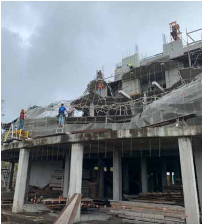
Fig. 3: Adding mesh to armature
