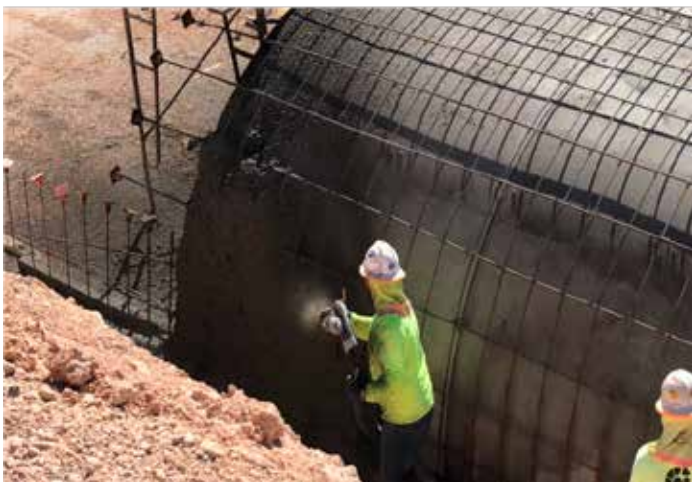
Fig. 8: Wrong angle shooting results in surface waviness
