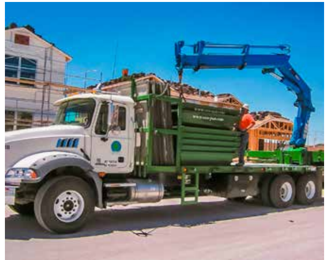
ECO-PAN crane truck unloading pump pans at a residential site
