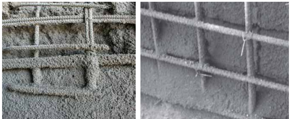
Fig. 6: Sandy or dull, opaque surface during placement
