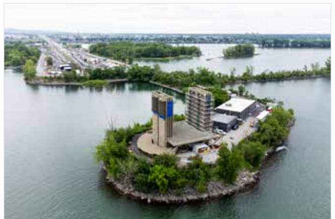
Fig. 2: Ventilation towers of the Louis-Hippolyte-La Fontaine tunnel. Photo credit: La Presse (2024).
