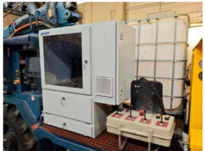
Fig. 1: Retrofitting the control system on an existing machine
