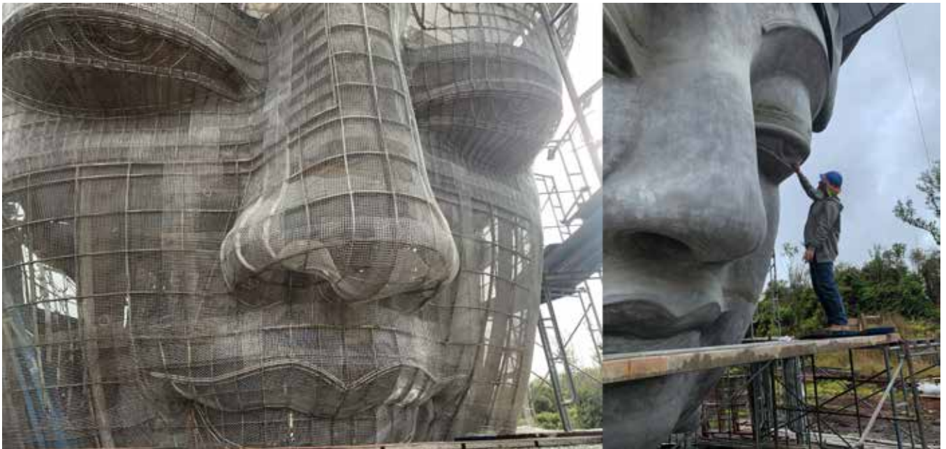
Fig. 5: Armature with mesh and 0.375 in. steel rods for better definition and finished mortar layer
