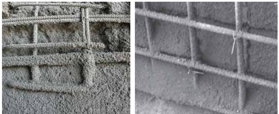
Fig. 6: Sandy or dull, opaque surface during placement
