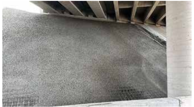
Fig. 5: Finished shotcrete wall with uniform texture and proper compaction for structural slope stabilization
