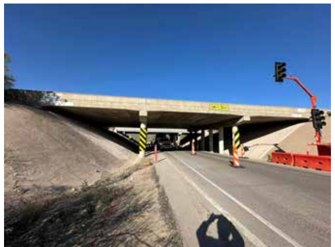
Fig. 6: Completed shotcrete slope protection under a highway overpass for long-term erosion control and durability
