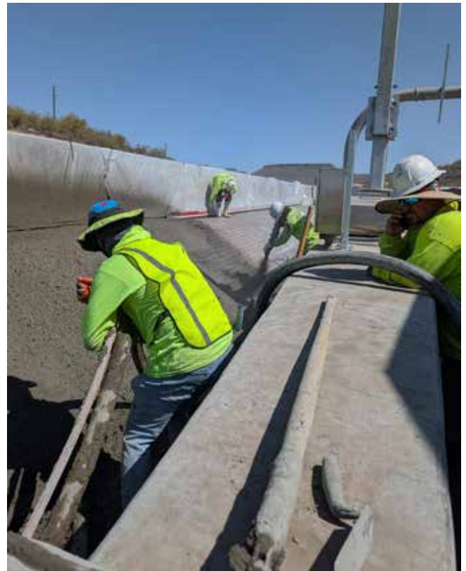
Fig. 3: Shotcrete crew placing concrete on reinforced slope protection along a highway embankment in Arizona
