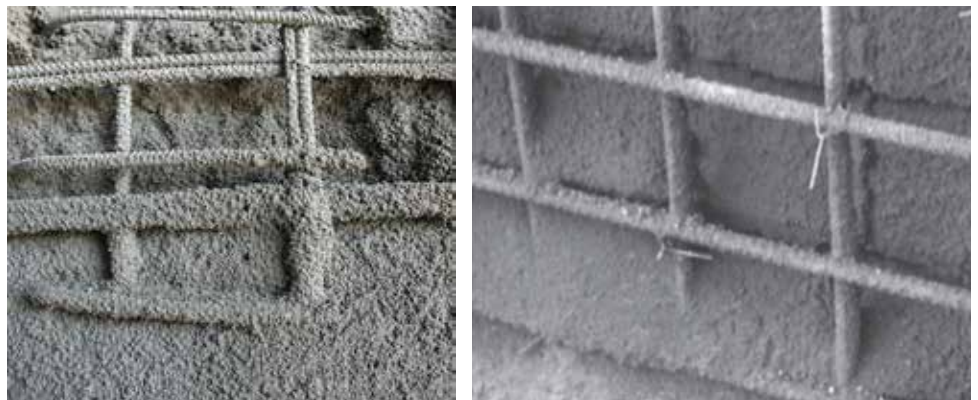
Fig. 6: Sandy or dull, opaque surface during placement
