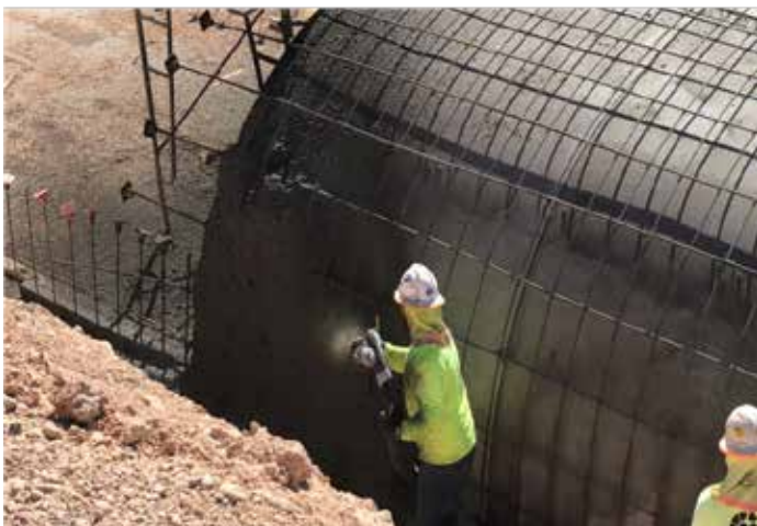
Fig. 8: Wrong angle shooting results in surface waviness
