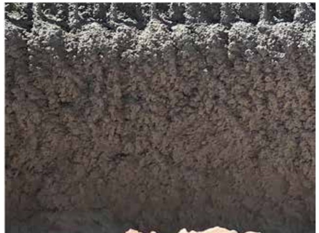
Fig. 8: Wrong angle shooting results in surface waviness
