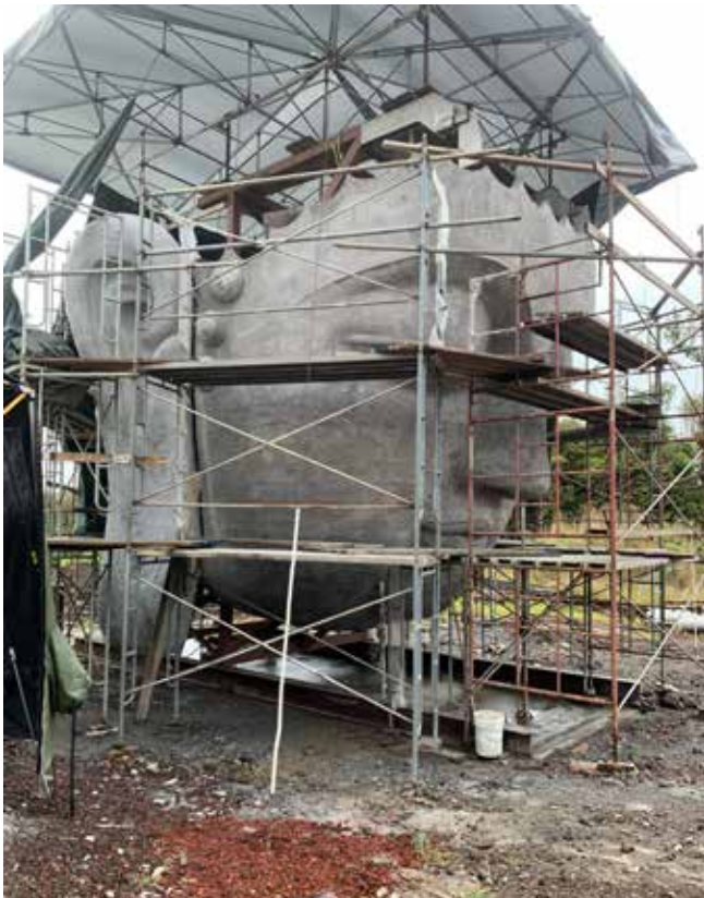
Fig. 2: Head on steel frame
