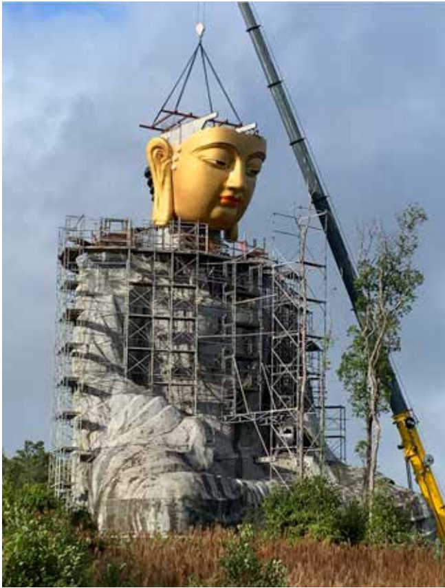
Fig. 7: Lifting parts of the head
