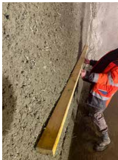
Fig. 9: An even shotcrete surface, achieved using the automated spraying system
