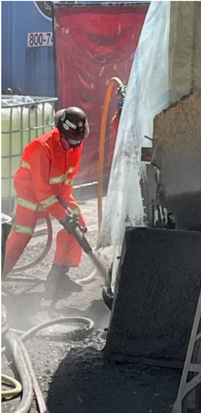
Fig. 1: Shooting panels for nozzleman certification on Newell Project, Santa Cruz, CA
