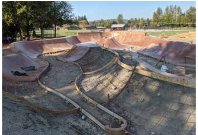
Fig. 2: Skatepark designers use earthwork to provide the shape and support of the concrete skating surface, then formwork is installed; photo courtesy of Grindline Skateparks, Inc.
