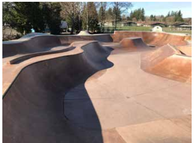
Fig. 4: Shotcrete is essential for achieving the smooth-flowing transitions in features such as bowls, pools, and banks; photo courtesy Grindline Skateparks, Inc.
