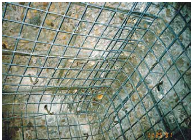
Fig. 1: HRSD James River WWTP damaged ordinary portland cement (OPC) concrete showing exposed aggregate, prepared with new rebar for initial SewperCoat® 2000 HS, 1991
