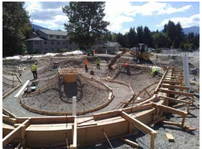
Fig. 3: Formwork for skateparks is custom-fabricated; photo courtesy Grindline Skateparks, Inc.
