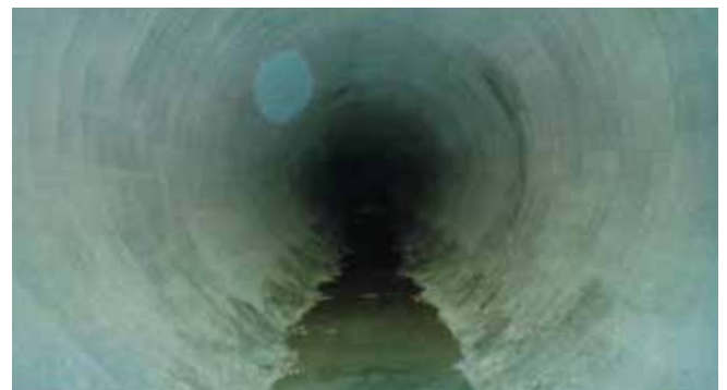
Figs. 3 & 4: Finished shotcrete lining
