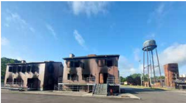
Fig. 5: Fondag® DG installed on all inner surfaces of fire academy burn buildings, still in service, 1999 and 2012
