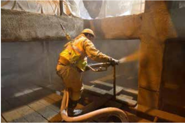
Fig. 3: Grit Chambers, Blue Plains Advanced WWTP, SewperCoat® 2000 HS, 2018
