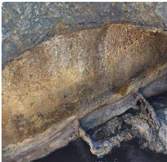
Fig. 2: HRSD James River WWTP inspection in 2022, still performing after 31+ years without additional rehabilitation, SewperCoat® 2000 HS
