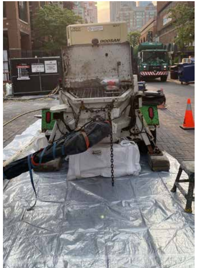
Fig. 5: Installing a 'Python' cover will confine concrete within the cover in the event of a rupture.
