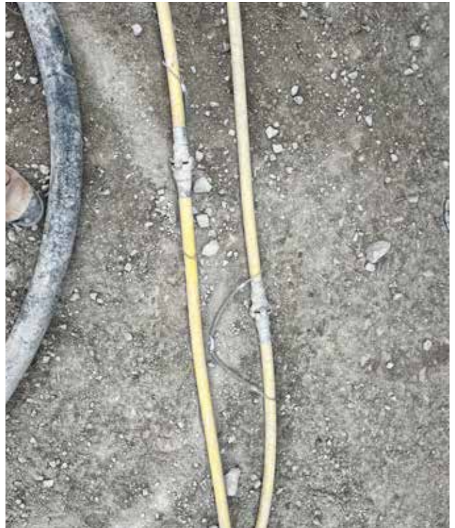
Figs. 1 & 2: Whip checks installed on material and airlines to restrain them in the event of a disconnection.
