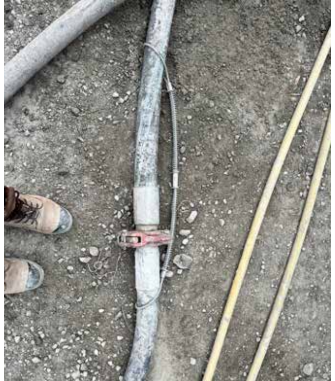
Figs. 1 & 2: Whip checks installed on material and airlines to restrain them in the event of a disconnection.
