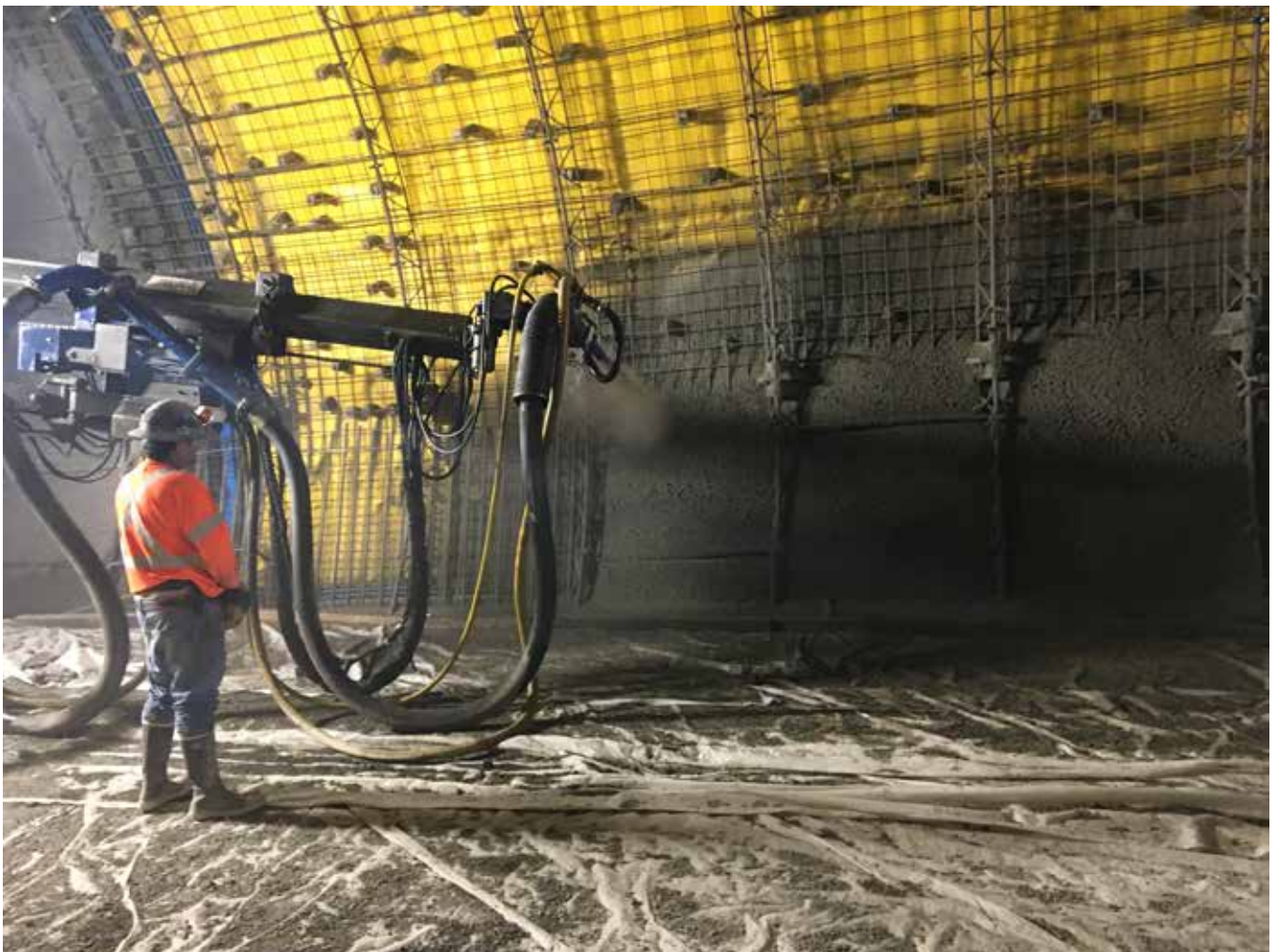
Fig. 2: Installation of SFL
