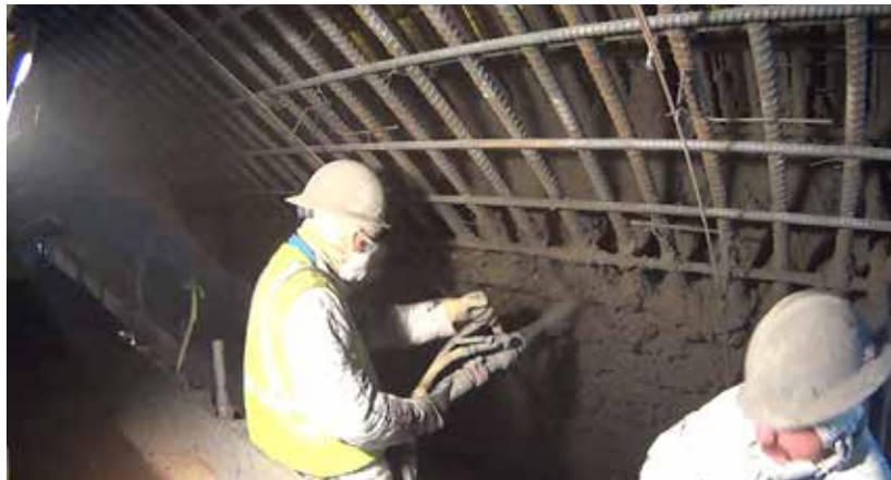
Fig. 4: Production Spraying
