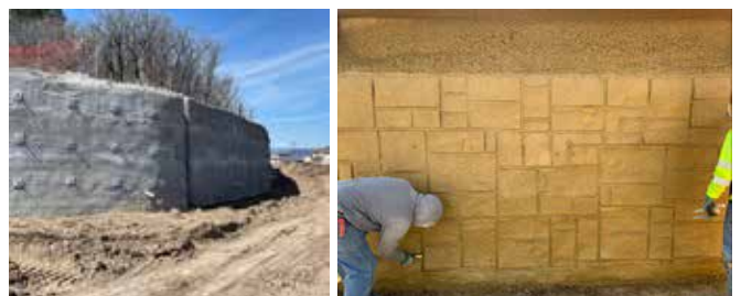
Figs. 3 and 4: Soil nail wall in progress
