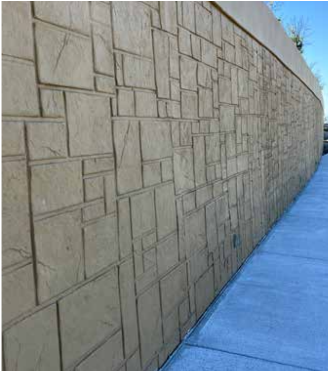
Fig. 4: Final carved soil nail wall
