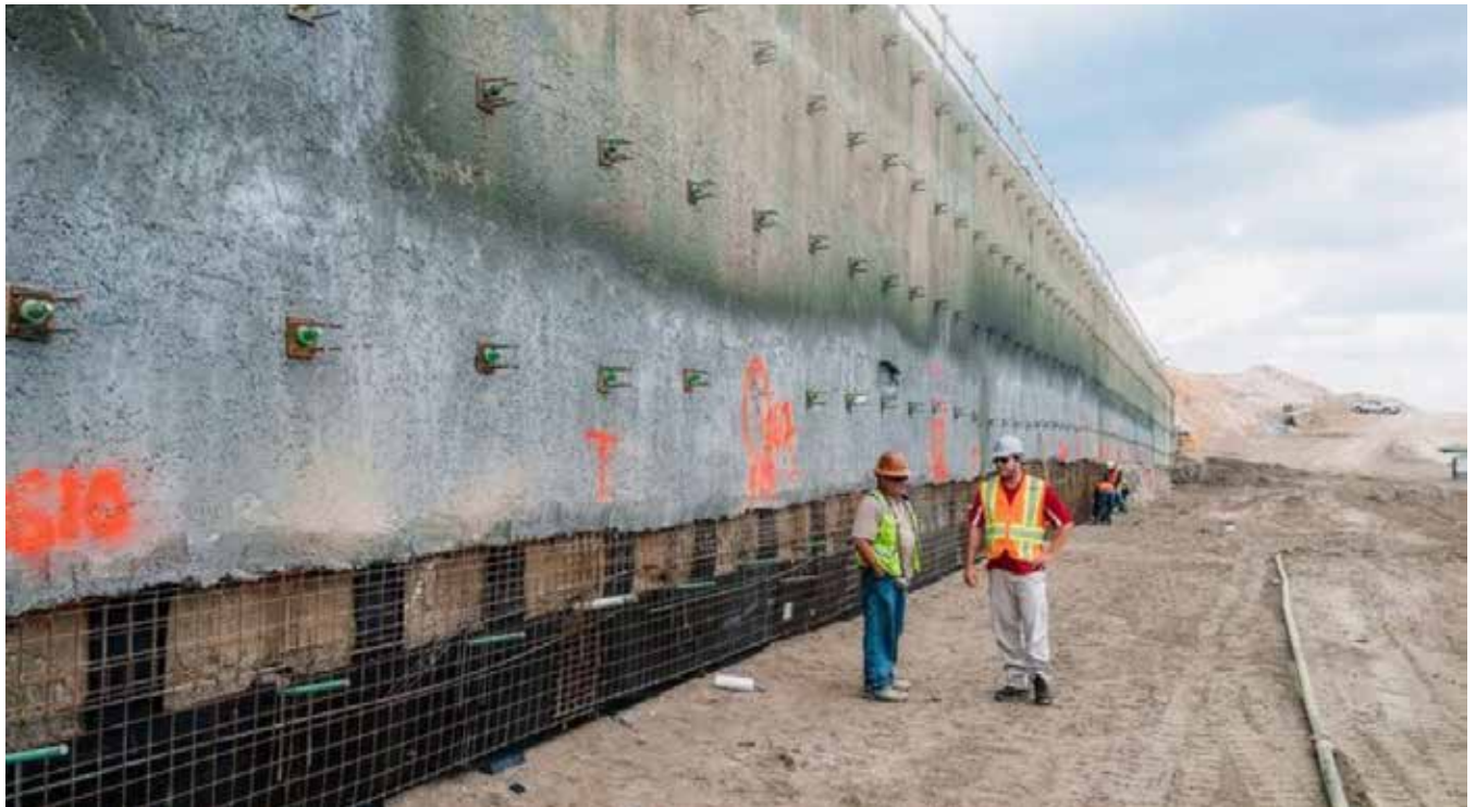
Fig. 2: Tall soil nail wall shot from top to bottom
