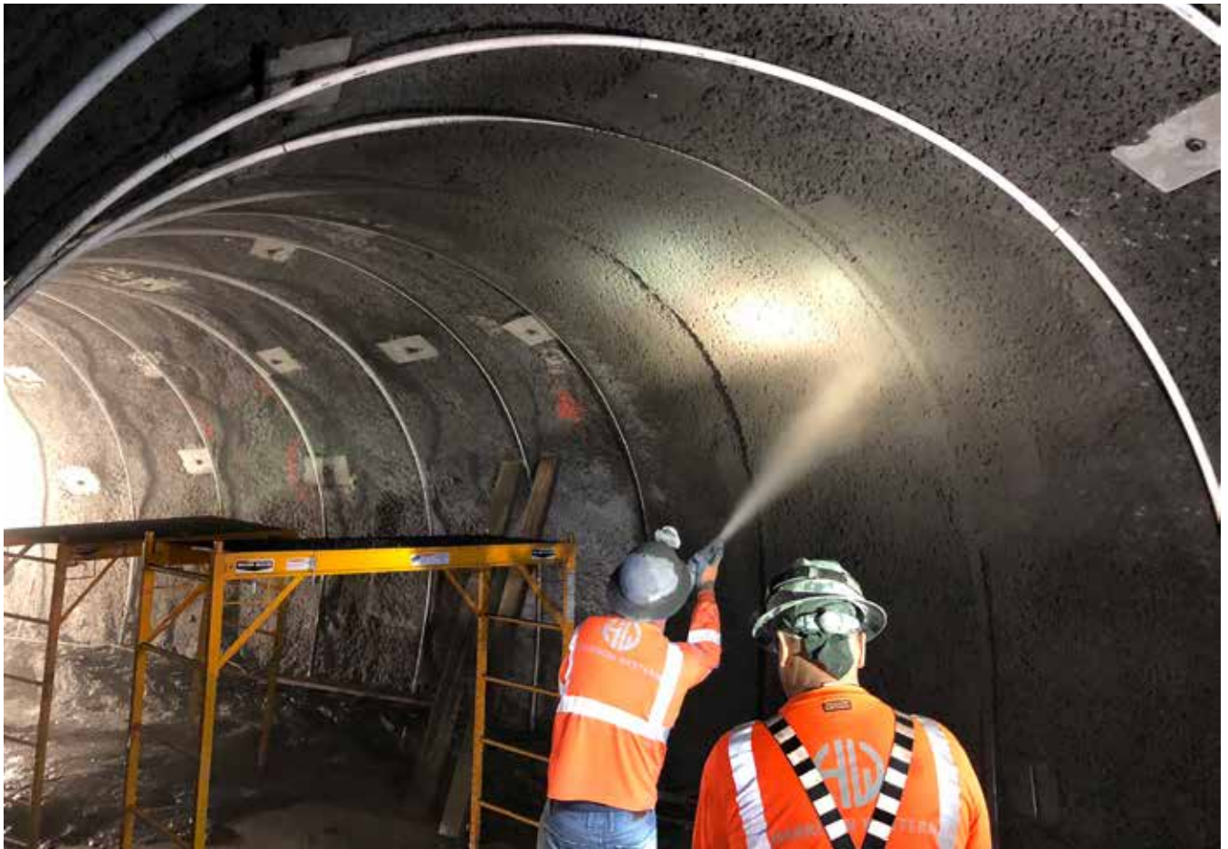
Fig. 4: Use guides for alignment and thickness
