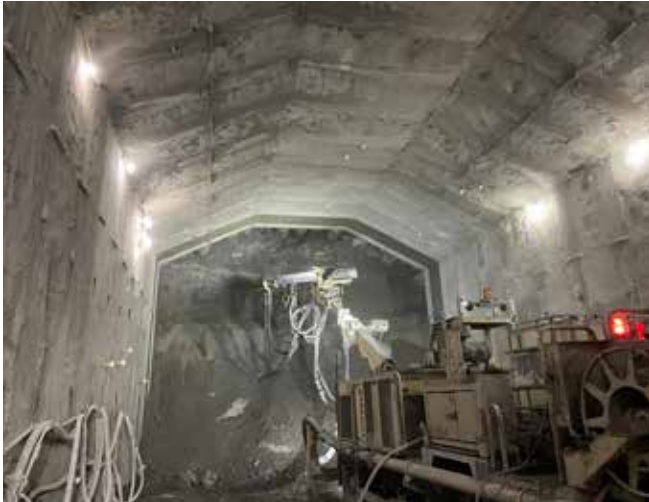
Fig. 3: Shotcrete robot (Normet Spraymec 8100 VC) applying flashcrete to the advanced top heading
