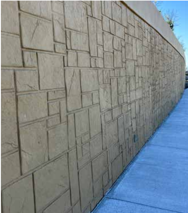
Fig. 4: Final carved soil nail wall
