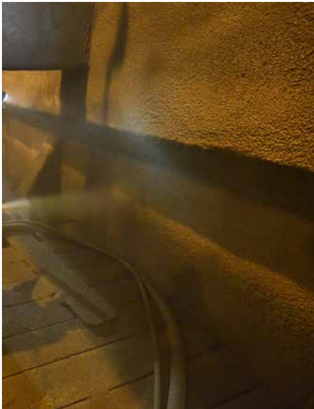
Fig. 4: Dry-mix application on wall
