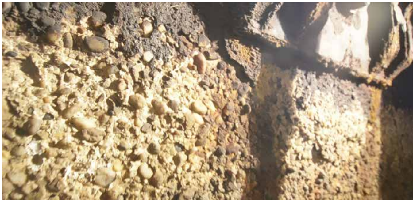
Fig. 1: Biogenic corrosion attacks concrete and steel
