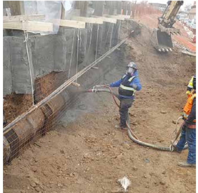
Fig. 1: Shooting soil nail wall with drainage behind
