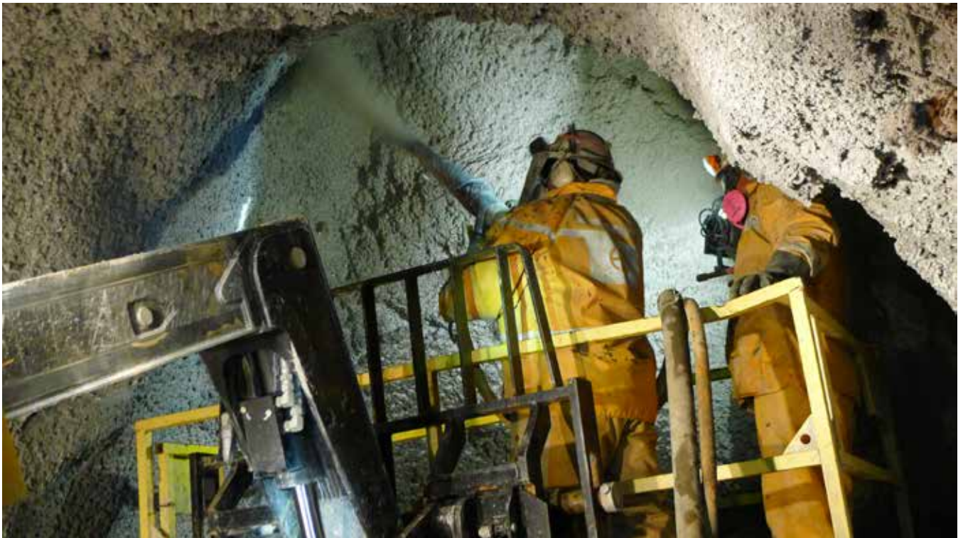
Fig. 3: Shooting underground on a platform with good light and ventilation
