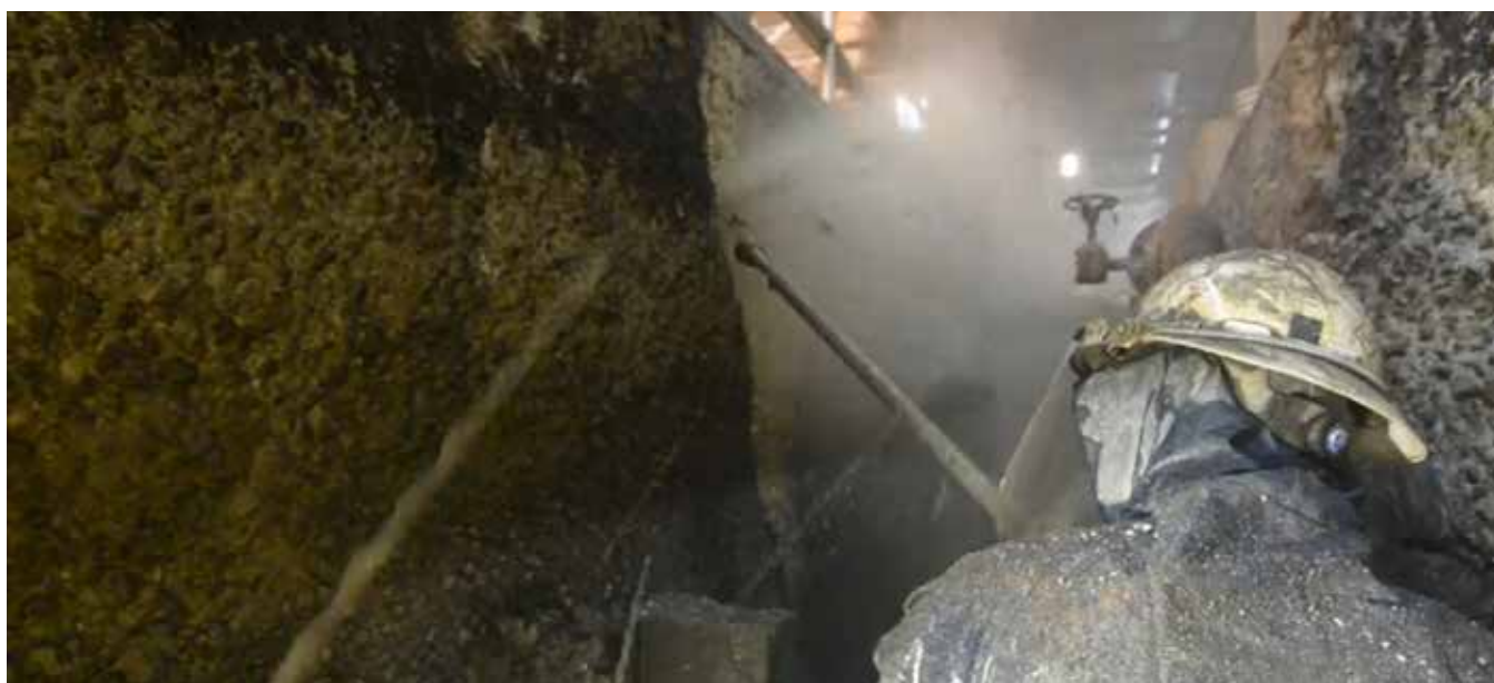
Fig. 3: Surface preparation via hydrodemolition
