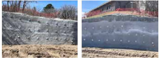
Figs. 1 and 2: Soil nail wall in progress
