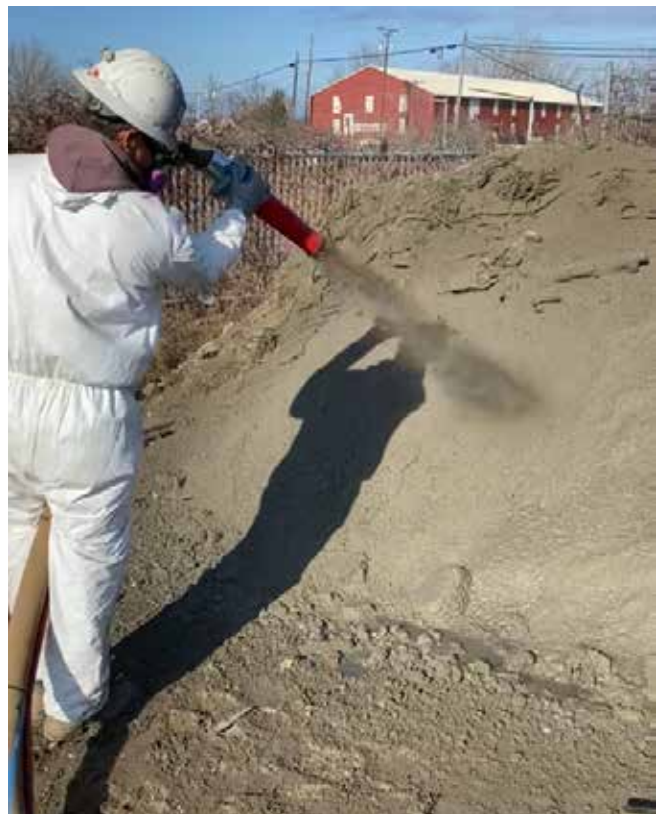
Fig. 2: Dry-mix shotcrete application
