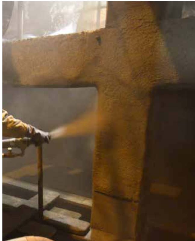
Fig. 5: Dry-mix application on column and beam
