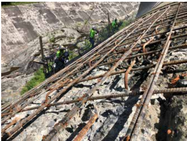
Fig. 2: Typical steel reinforcing: #5 (#16M) L-dowels at 2 ft (0.6 m) spacing with a #5 rebar at 1 ft (0.3 m) on center each way
