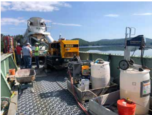
BELOW: Fig. 6: Shotcrete pumping and chemical dosing operation from the bridge overhead
