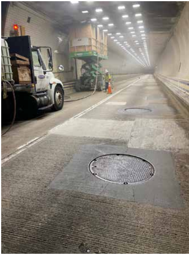
Fig. 3: Shotcrete placement in the tunnel
