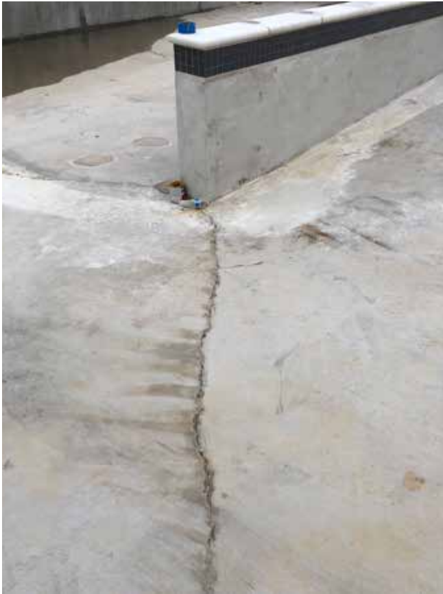
Fig. 5: Shrinkage cracks at reentrant corner.
