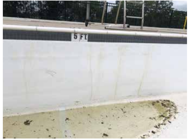
Fig. 5: Shrinkage cracks at reentrant corner.
