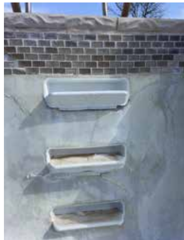
Fig. 8: Shrinkage crack at underwater light.
