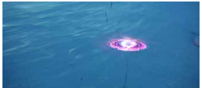
Fig. 8: Shrinkage crack at underwater light.
