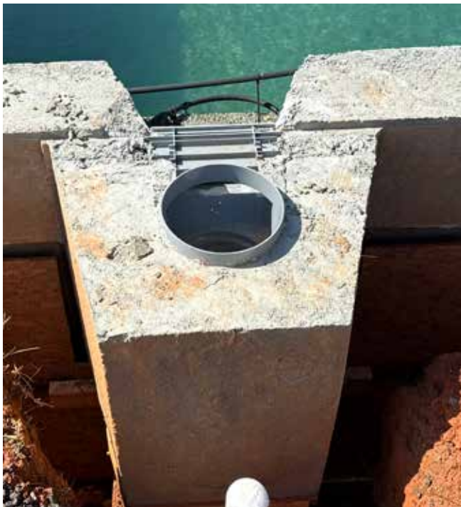
Fig. 5: After shotcrete placement during 28-day water cure.
