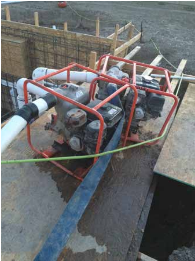
Fig. 4: Trash pumps around pool for dewatering with well points used to successfully drain ground water during construction phase.
