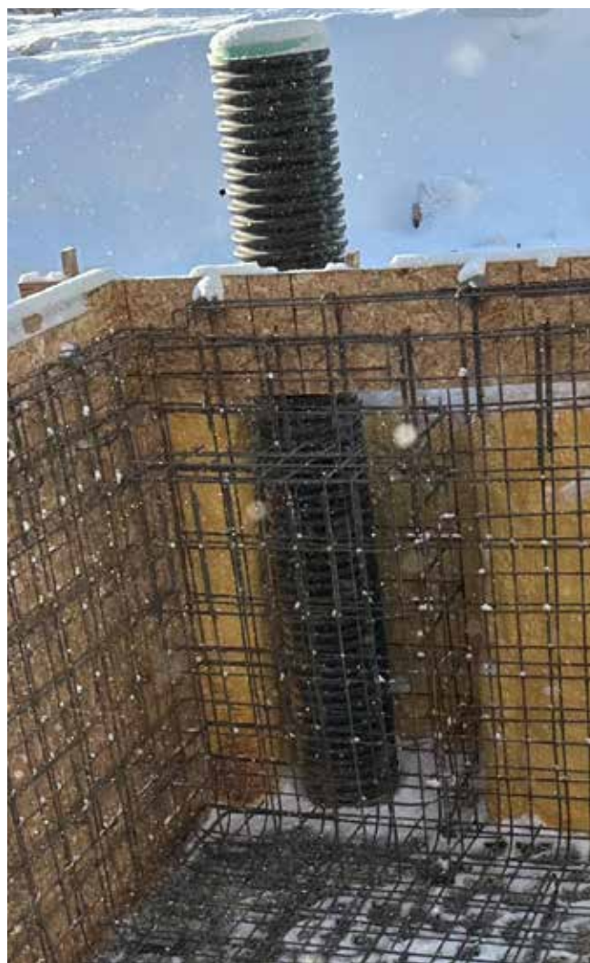
Fig. 2: Sump pump style pipe installed near pool base with pump inside removing ground water.
