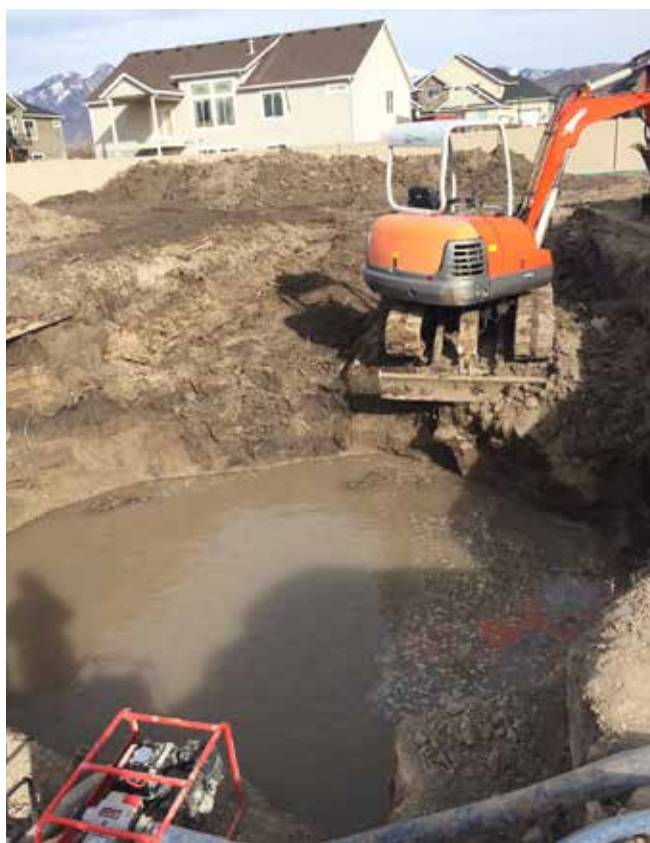
Fig. 1: A pool excavation in definite need of dewatering.
