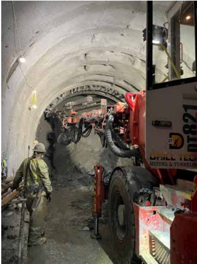
Two-boom jumbo installing pre-support spiles over steel set arches and shotcrete tunnel lining
