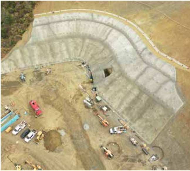
Aerial view of the 48,000 ft 2 (4500 m 2 ) soil nail & reinforced shotcrete portal and the beginning of tunnel excavation
