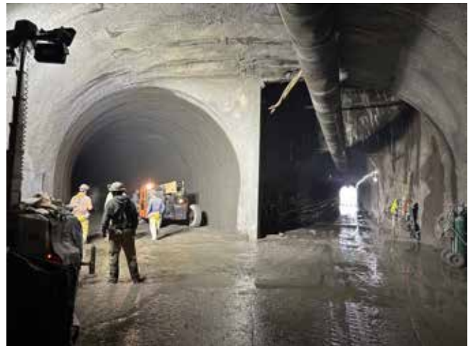
Looking into the Transition Zone bifurcation/intersection; comparison of complete smoothing shotcrete on left side and the in-progress right side which had yet to be completed
