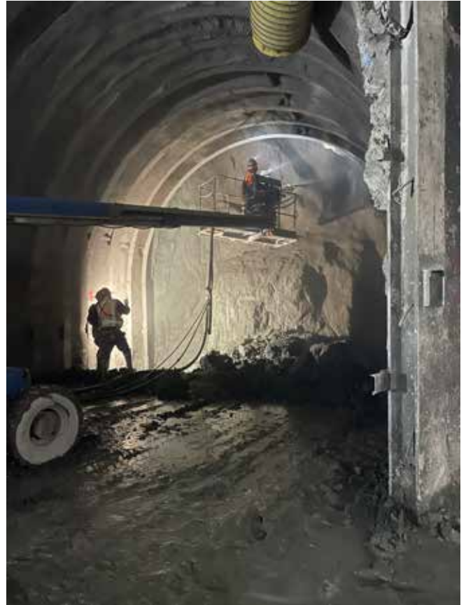
Tunnel Shotcrete placement via manlift and hand nozzle in 24 ft diameter tunnel
