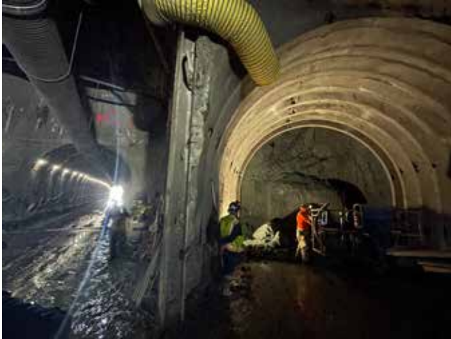
Photo taken viewing tunnel bifurcation/intersection area, shotcrete liner visible in both tunnels
