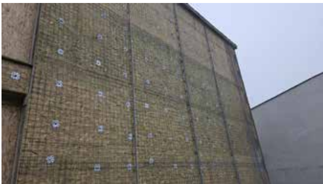
Reinforcement, expansion joints, and preparation for shotcreting
