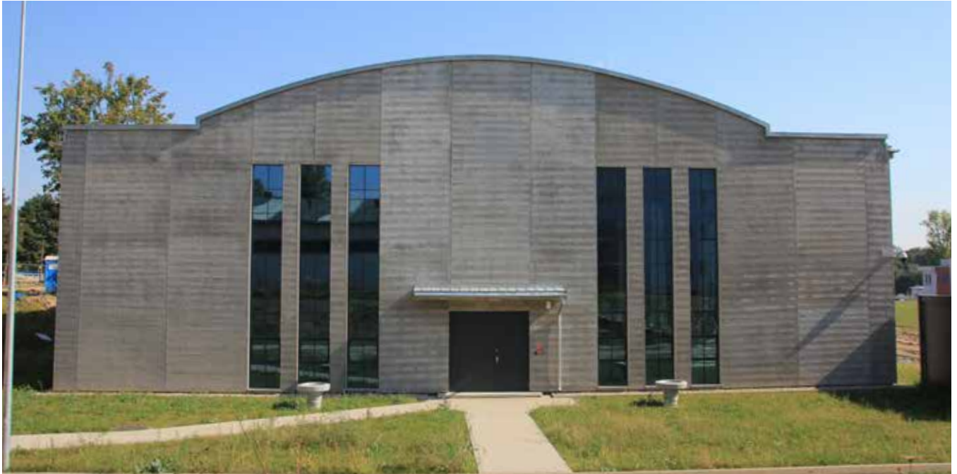
Façade after work completion
