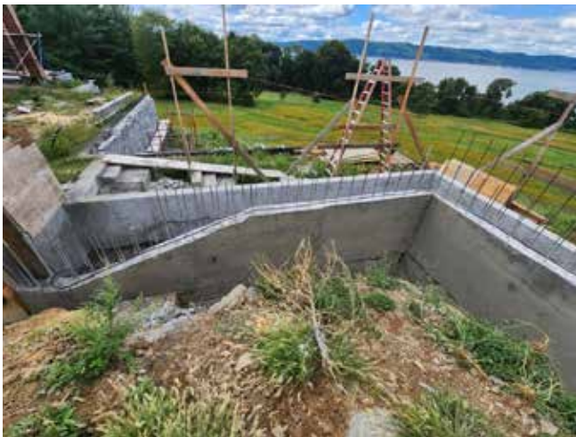
Fig. 4: Poured foundation formed for on grade support of shotcreted pool
