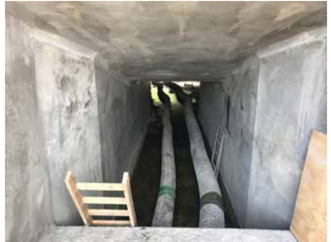
Shotcrete for box culvert lining walls
