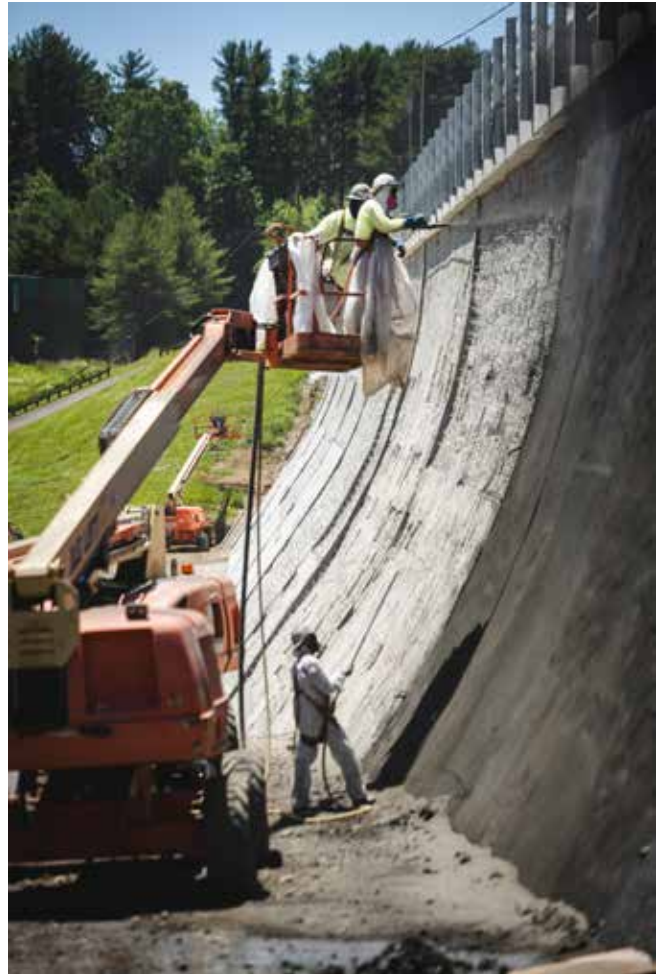
Fig. 5: Downstream shotcrete application
