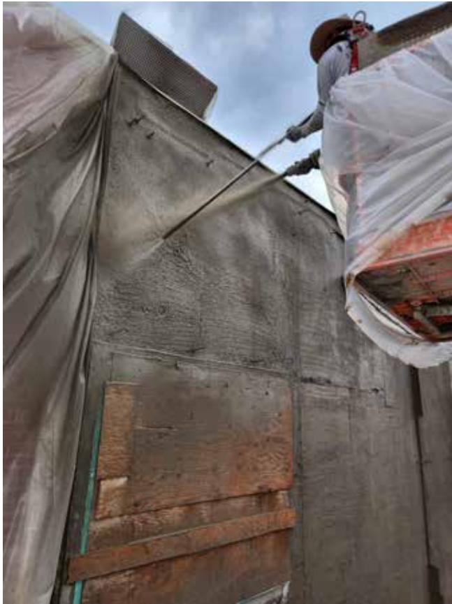
ABOVE: Fig. 1: Maintaining a clean surface with an air lance
