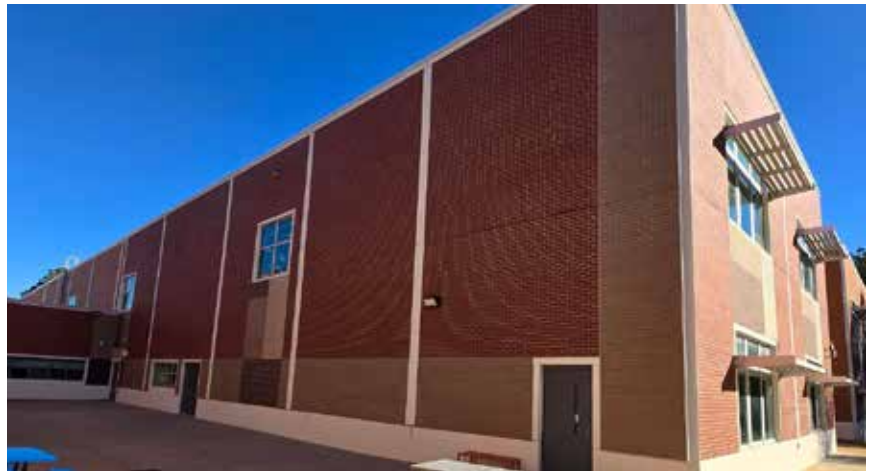
Fig. 8: Finished walls after cladding
