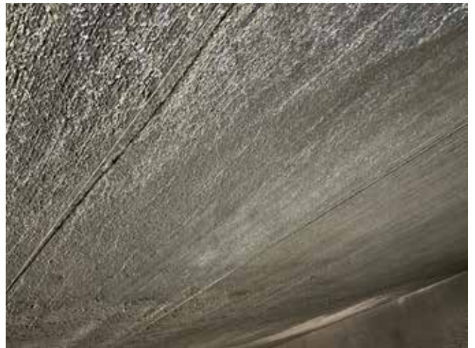
Final broom finish of the draft tube ceiling modification
