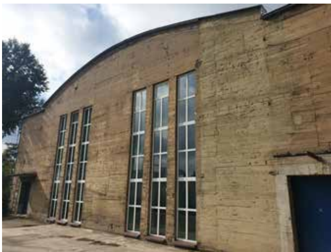
Façade of Rapid Filter Building before renovation
