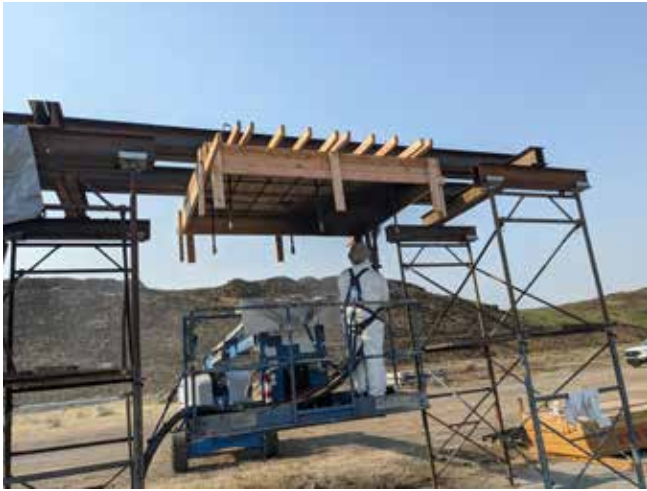
Shotcreter shooting the full-scale mock-up
