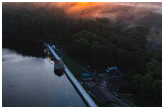
Fig. 2: Hemlock Dam upstream and gate house repair area
