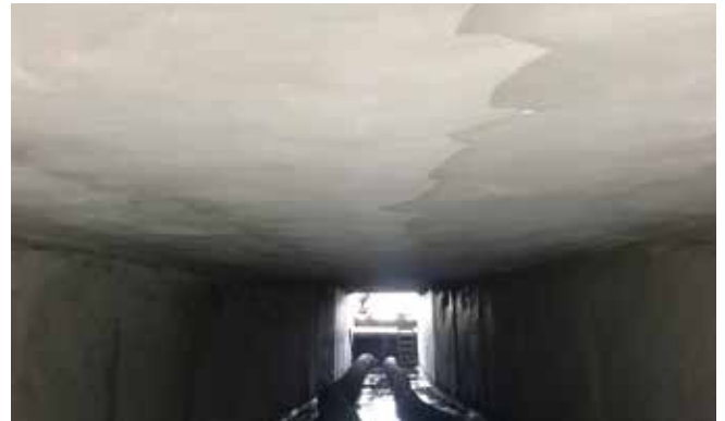
Shotcrete for box culvert lining ceiling
