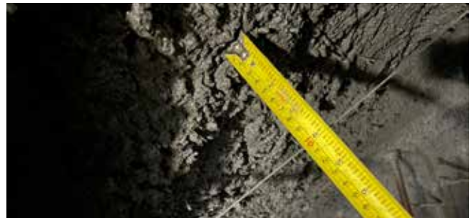
Layer thickness was controlled to a maximum of 4" using steel piano wire
