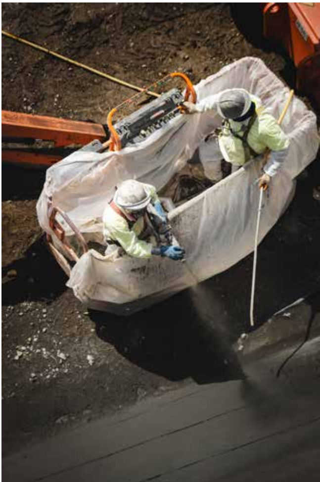
Fig. 4: Shotcrete application from 80 ft (24 m) man lift
