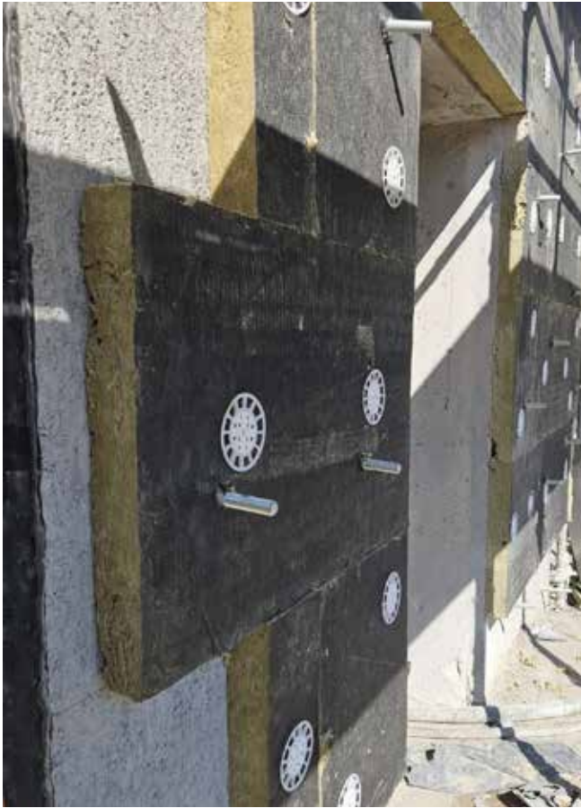
Installation of anchors and building insulation
