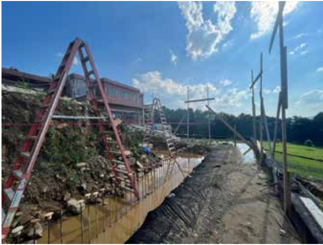
Fig. 3: Original soils and elevations to form and to work up to
