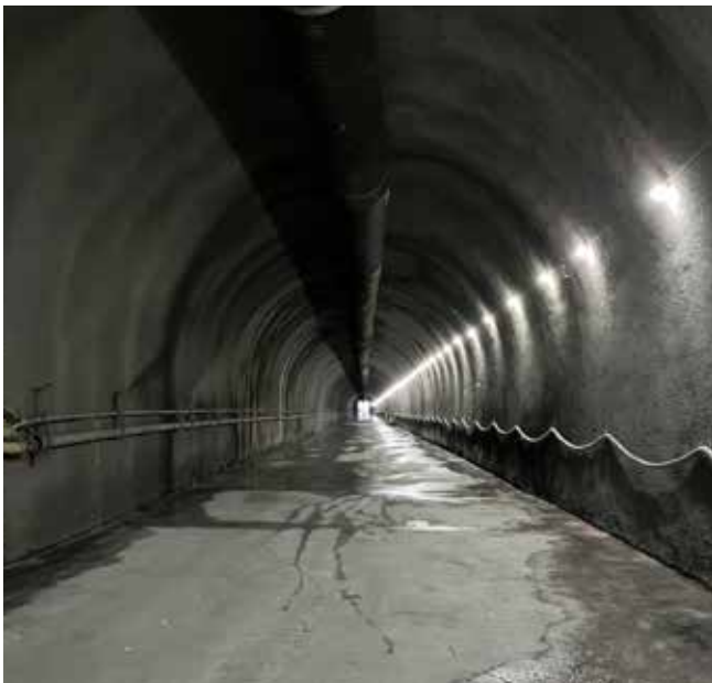
Smoothing shotcrete interior surface complete looking out of tunnel toward the portal
