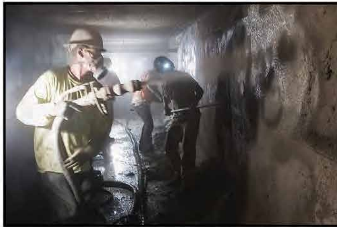
REED's portable SOVA Gunite Machine is perfect for small concrete repair jobs
