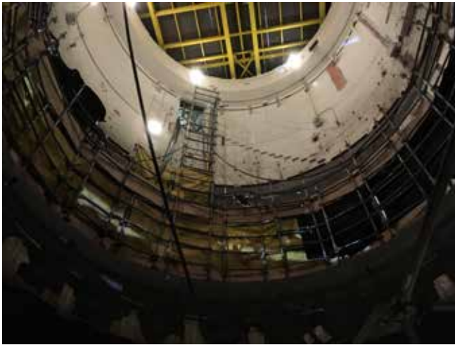
Shaft for a turbine unit
