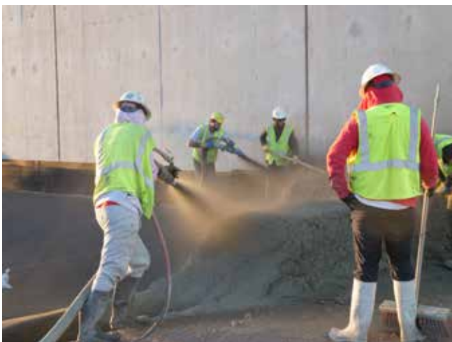
Shotcrete Oil Pit Installation for Transformer Switchgear: Workers installing a robust oil containment pit using shotcrete, designed for safety and environmental protection in industrial applications.
