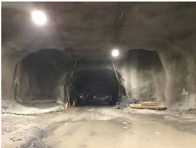
Figure 9: Excavation at the platform level excavation
