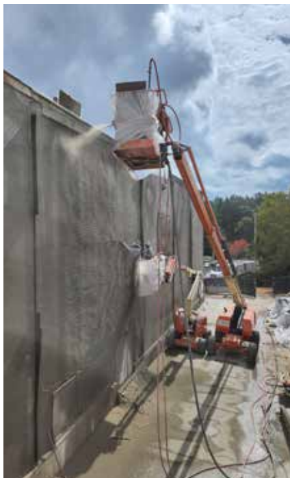
ABOVE: Fig. 1: Maintaining a clean surface with an air lance
