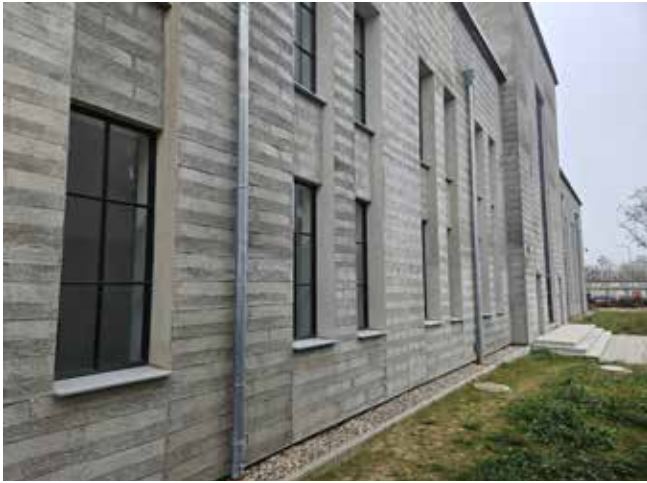
Façade after work completion
