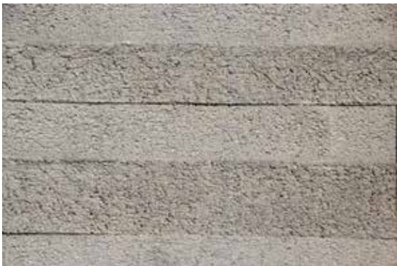
BELOW: Final effect of formwork
