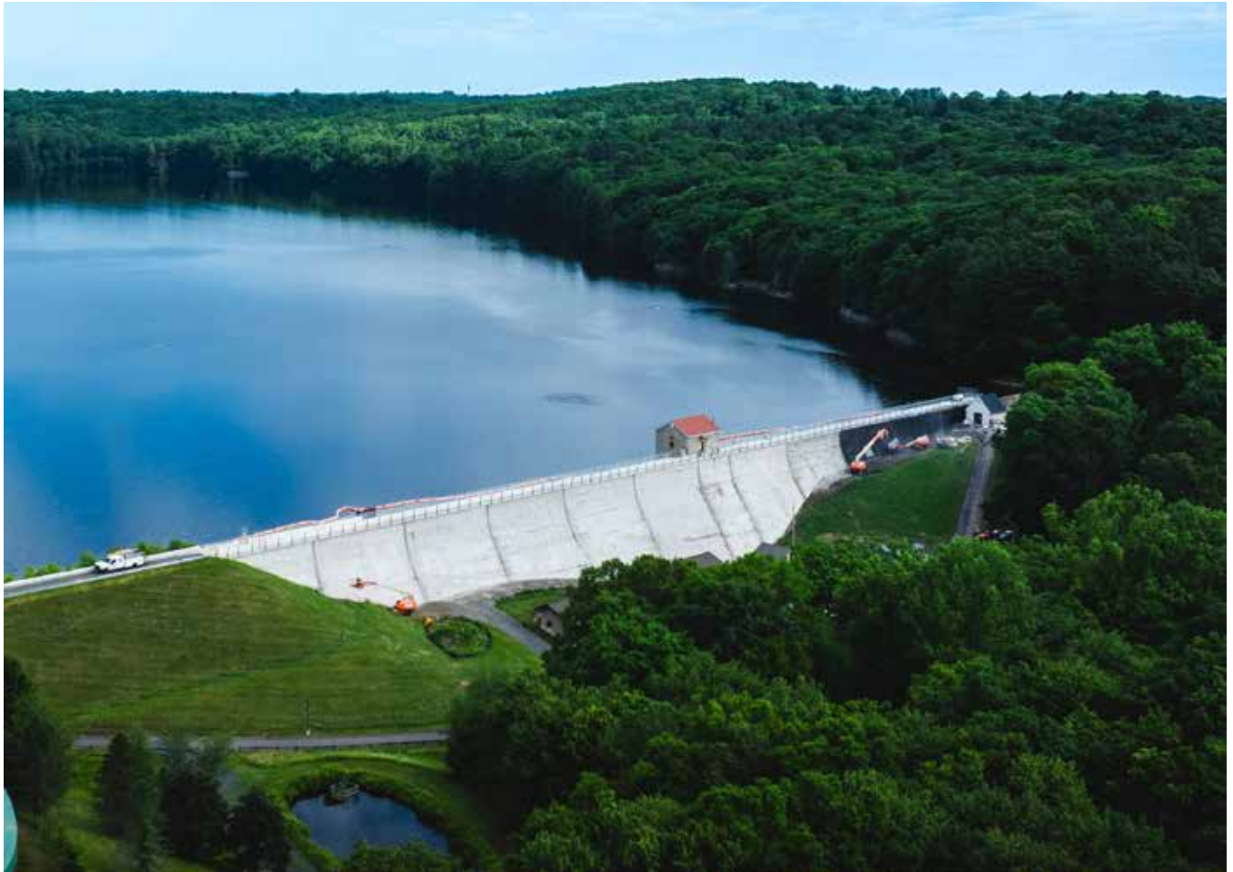
Fig. 1: Hemlock Dam downstream repair area
