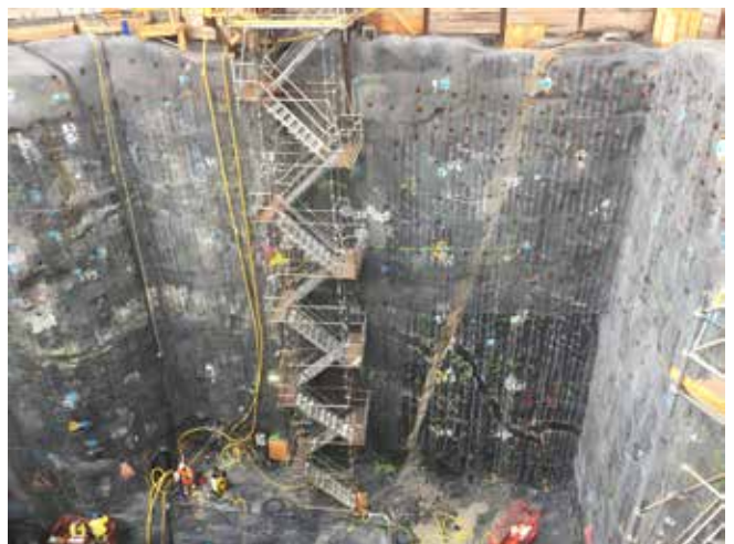
BOTTOM 2: Fig. 7: Photos of the waterproofing membrane spraying on the shaft walls
