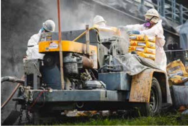
Fig. 3: Wet-mix pump with mixer using prepackaged repair mortar
