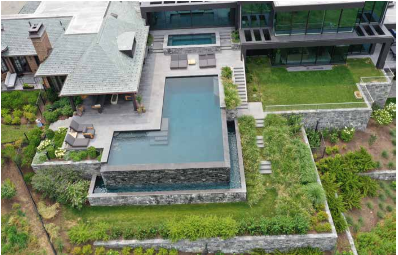
Fig. 8: Drone footage showing line and grade balance and symmetry
