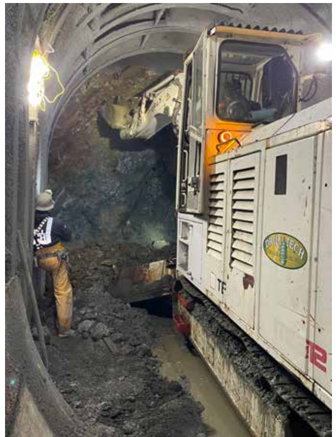
Tunnel excavation progressing ahead of steel arch set and shotcrete liner
