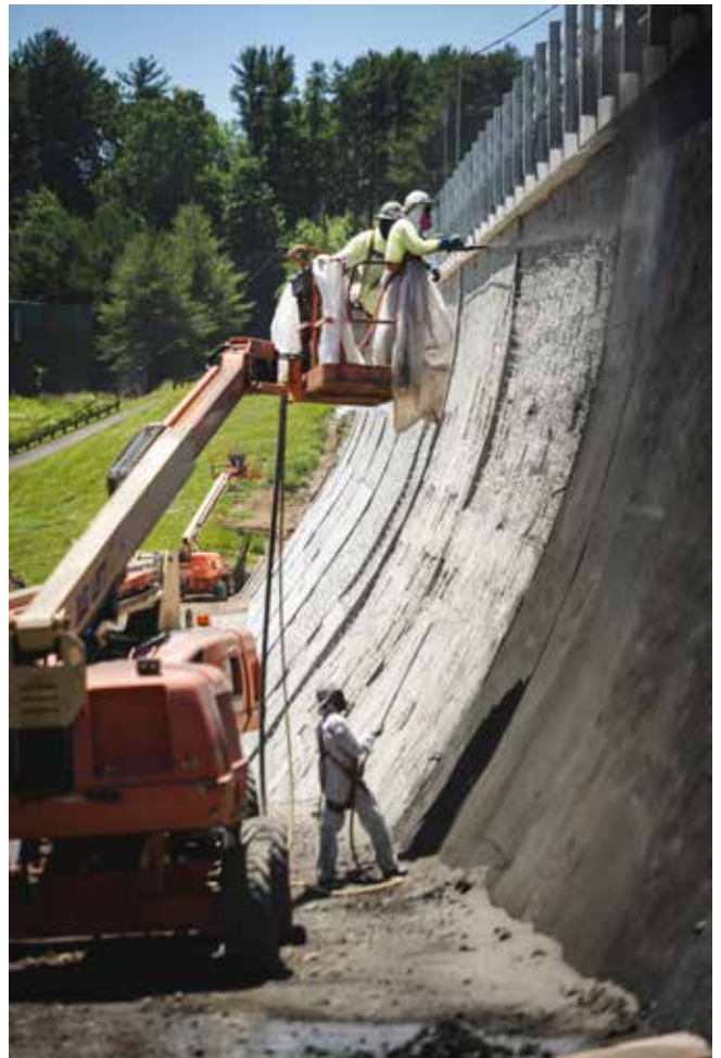
Fig. 5: Downstream shotcrete application
