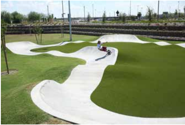
Eastmark Skatepark in Mesa, AZ: BAM Shotcrete played a key role in constructing this modern skatepark, delivering expertly crafted concrete tracks and smooth surfaces for skaters to enjoy.
