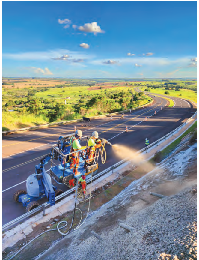
Fig. 8: Application of shotcrete using an articulating boom lift.
