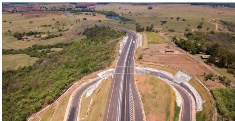
Fig. 2: Aerial view of roadside slope.
