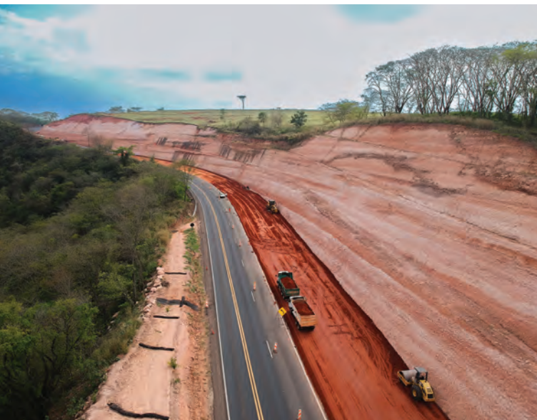
Fig. 3: Excavation and slope process for highway expansion.
