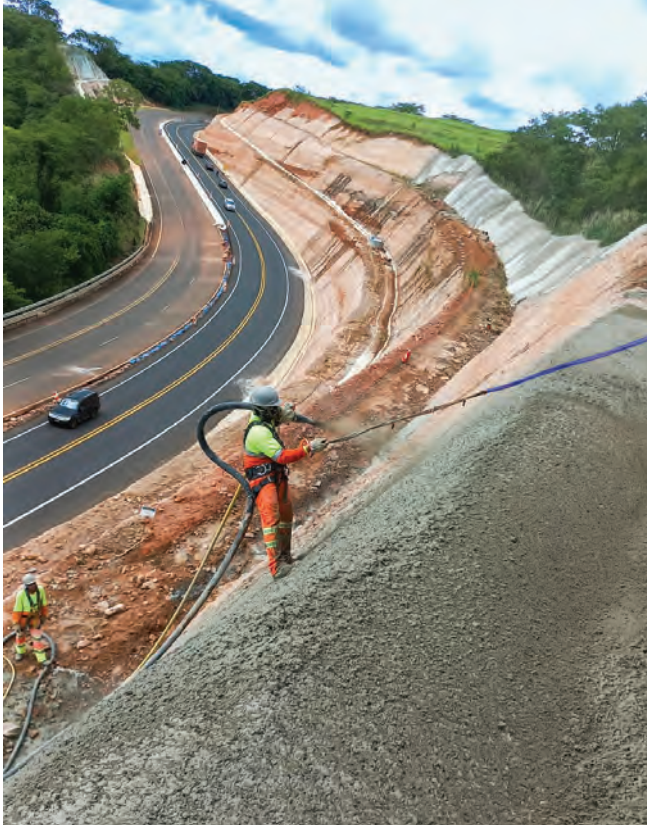
Fig. 7: Application of shotcrete using the rappelling technique.
