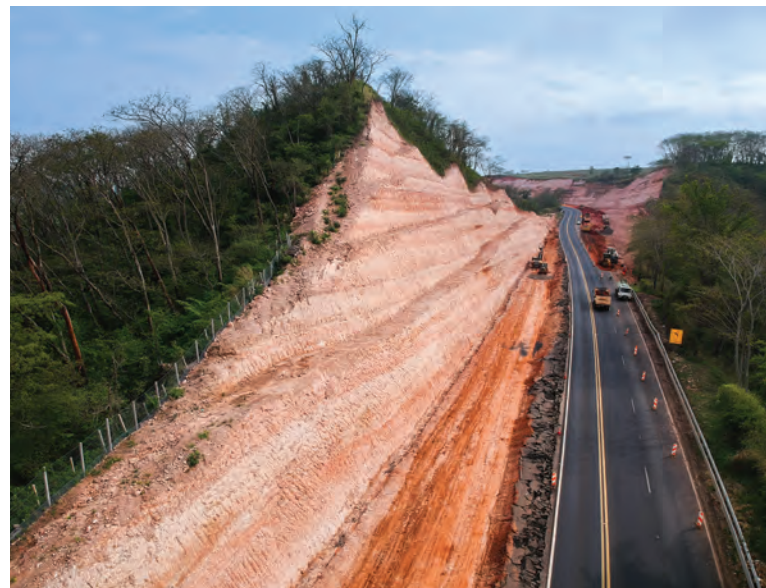
Fig. 4: Additional view of the excavation and slope process.
