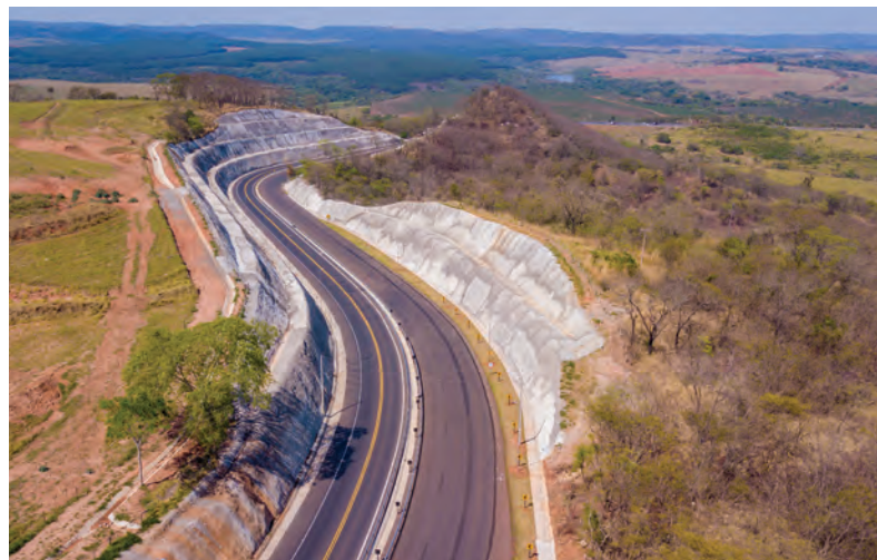
Fig. 13: Another aerial view of the completed slope.
