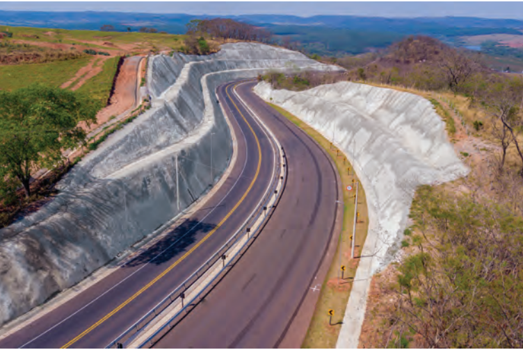
Fig. 10: Slope after shotcrete application.
