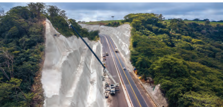
Fig. 5: Application of shotcrete from a man basket using a crane.
