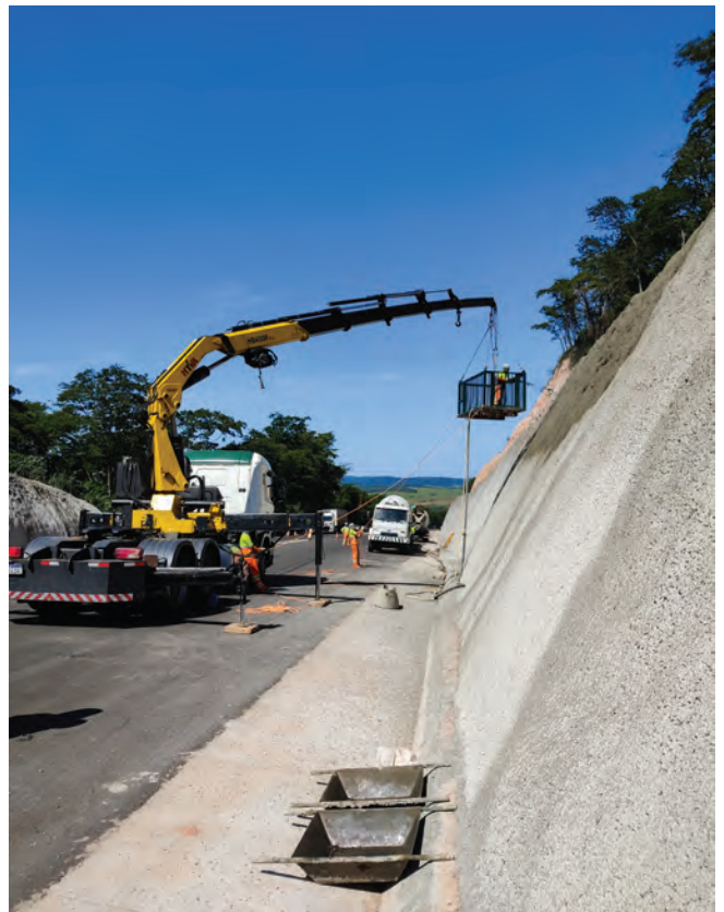
Fig. 9: Application of shotcrete using a truck-mounted crane.
