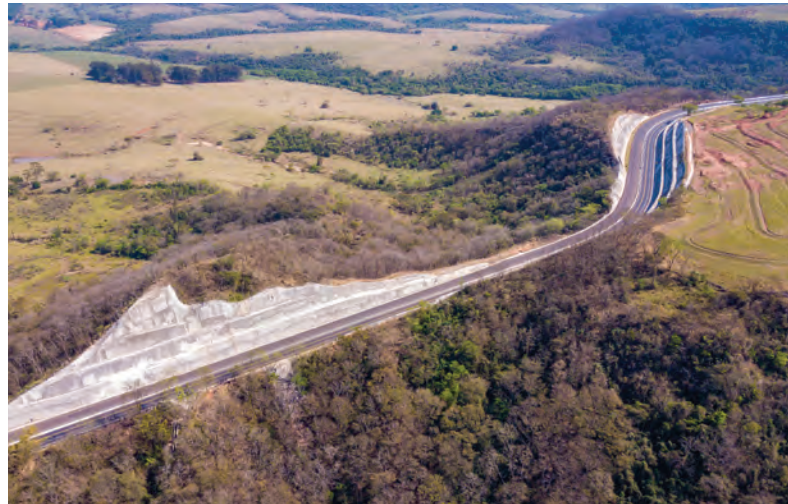
Fig. 12: Aerial view of the completed slope.
