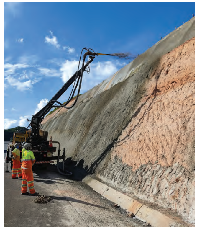
Fig. 6: Application of shotcrete using a shotcrete placing robot.
