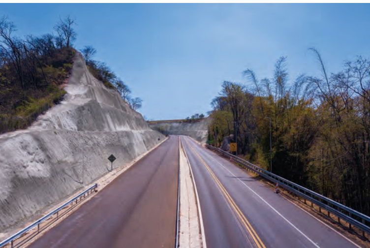
Fig. 11: Another view of the slope after shotcrete application.
