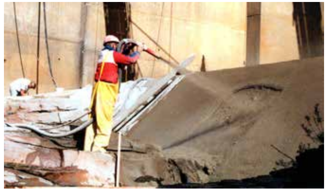
Dry Process Shotcrete repairs on the base of a dam in central Pennsylvania. Conveying and efficiently placing material is one of many hidden advantages of using shotcrete.
