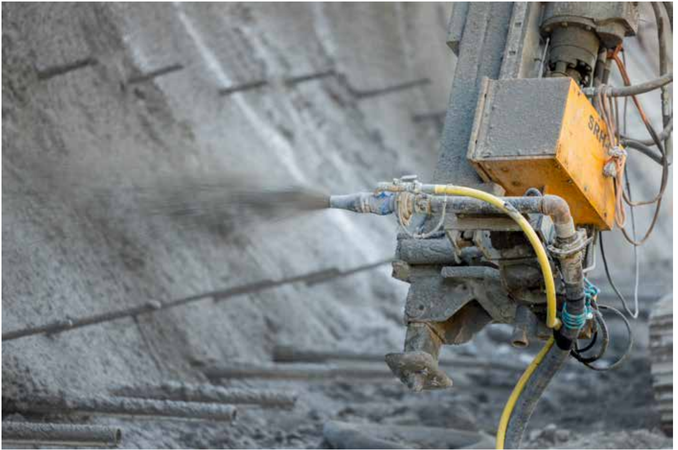
The remotely manipulated nozzle spraying concrete along the 1-65 interstate corridor.
