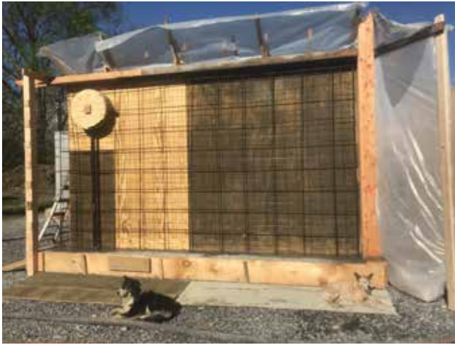
Wall formwork with Kahncrete dog inspectors Lex & Heyla.
