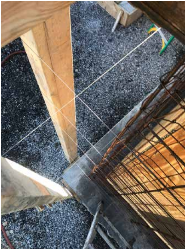
Guide wires set to define outside corner of the wall.
