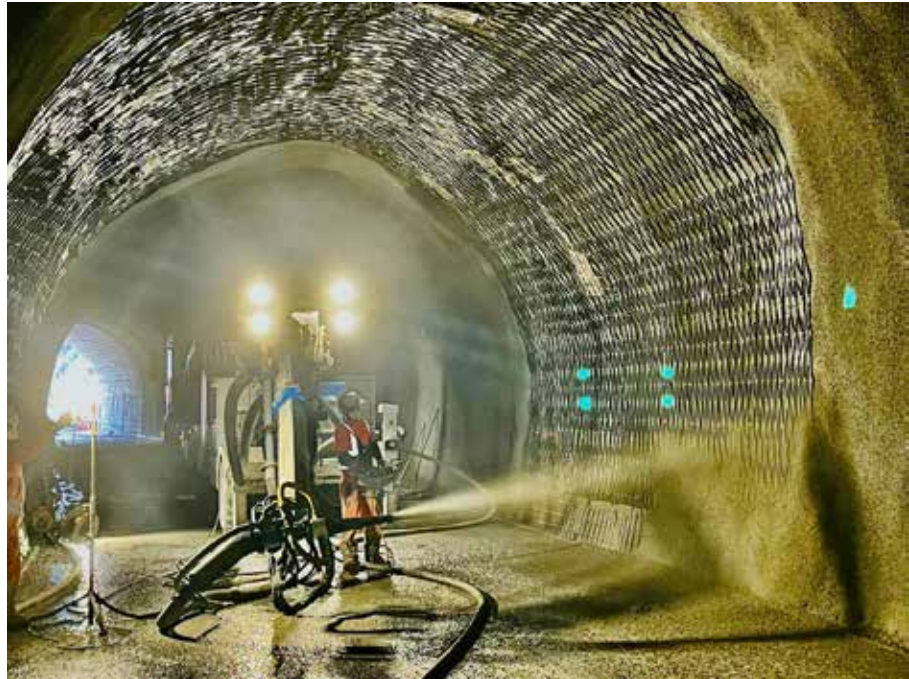
Fig. 6: Solution 1a application: a - LEFT) Dolenco Drain is covering the entire surface of the repaired area and secures permanently against water pressure (Tuscarora Mountain Tunnel); b - ABOVE) Renovating seeping road tunnel (La Tzoumaz, Switzerland)
