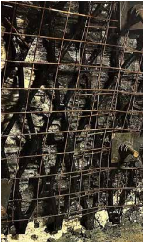
Fig. 8 (LEFT): Allowing shotcrete placement with water inflow using Dolenco Drain directly on the rock surface, with anchored wire mesh. Toronto, Canada
