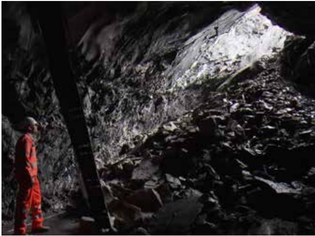
Fig. 2: Collapsed tunnel
