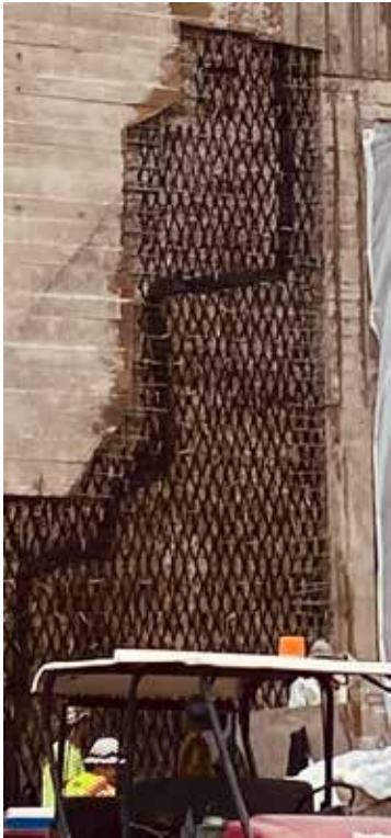
Fig. 6: Solution 1a application: a - LEFT) Dolenco Drain is covering the entire surface of the repaired area and secures permanently against water pressure (Tuscarora Mountain Tunnel); b - ABOVE) Renovating seeping road tunnel (La Tzoumaz, Switzerland)
