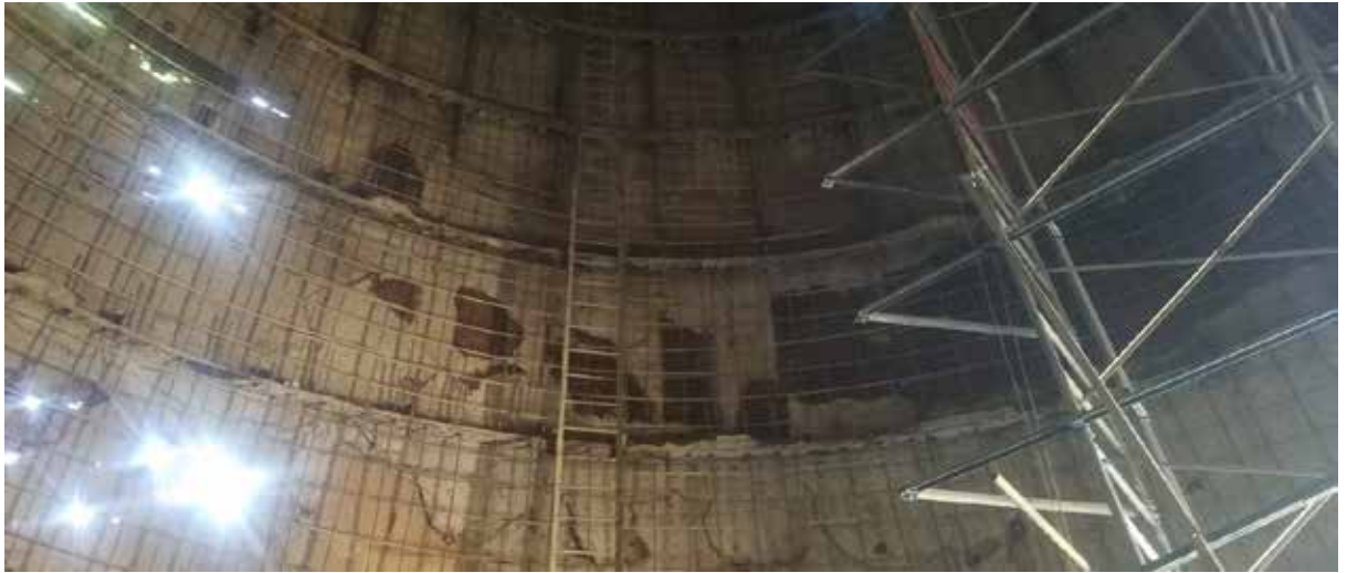
Steel Silo Lining Project
