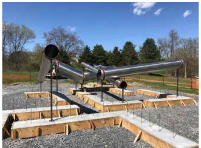
Mirror finished stainless steel pipes from Poland, suspended in place before shotcrete application.
