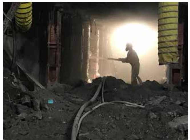
Fig. 6: Cedarvale Station, Eglinton West Intersection, courtesy of HC Matcon Inc.
