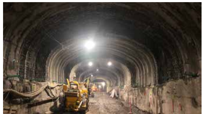
Fig. 7: Solution 1b application: a - ABOVE) Dolenco Drain was used to control the water by installing behind the shotcrete smoothing layer (Réseau Express Métropolitain); b - BELOW) Repair of railway tunnel (Canfranc, Spain).
