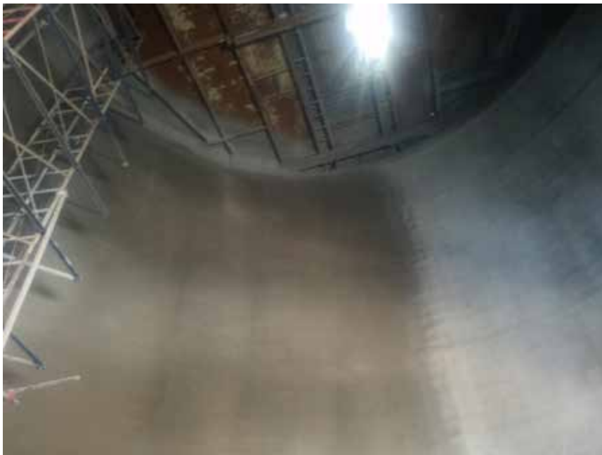
Steel Silo Lining Project
