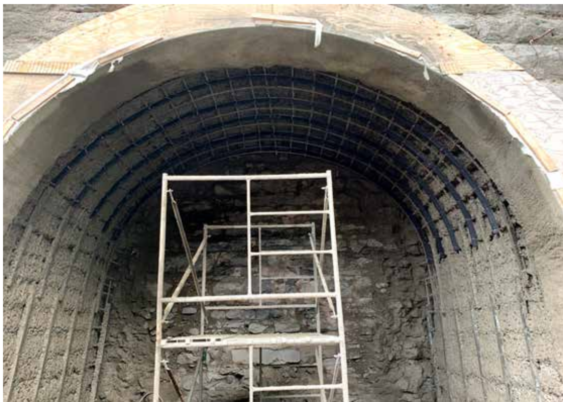
Nashville Tunnel Mid-Construction
