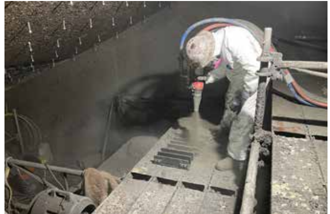
Shooting into an end beam form. Photo credit PCiRoads, LLC.
