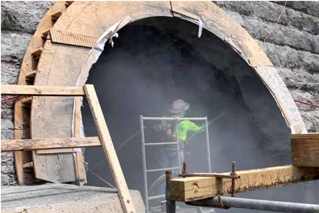
Nashville Shotcrete Application
