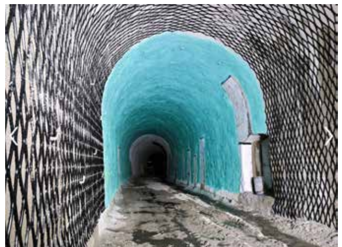
Fig. 7: Solution 1b application: a - ABOVE) Dolenco Drain was used to control the water by installing behind the shotcrete smoothing layer (Réseau Express Métropolitain); b - BELOW) Repair of railway tunnel (Canfranc, Spain).
