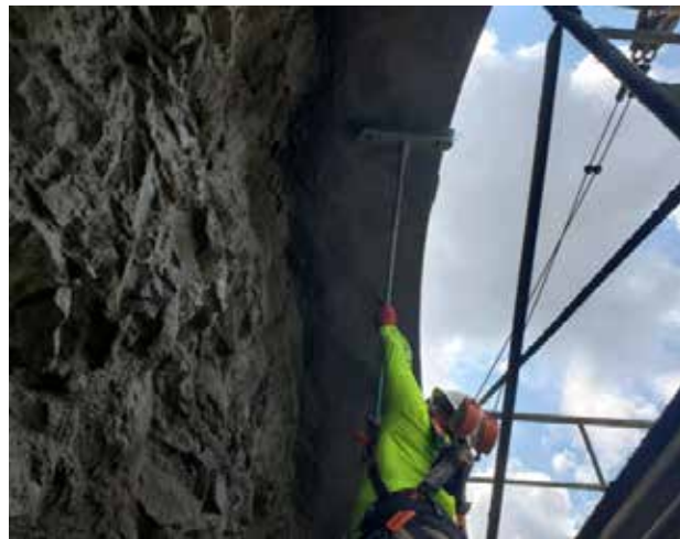
Nashville Soft Broom Finish Shotcrete
