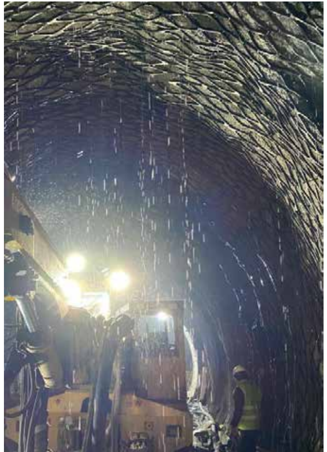
Fig. 1: Some of examples of water pressure effects: a) Leaking tunnel in waterproofing process (ABOVE); b) Icicles causing damage to a concrete structure (BELOW) (photo: Washington State Dept. of Transportation).
