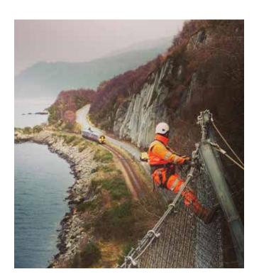
(DCP) anchors drilled into bedrock to fix the shotcrete wall in position. Geo-Rope Ltd used a combination of long reach plant and rope access A-frame to achieve this.
