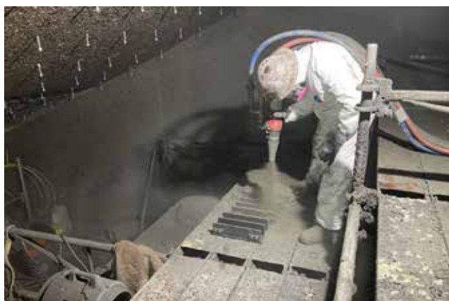
Shooting into an end beam form. Photo credit PCiRoads, LLC.
