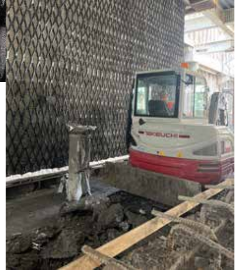
Fig. 8 (LEFT): Allowing shotcrete placement with water inflow using Dolenco Drain directly on the rock surface, with anchored wire mesh. Toronto, Canada
