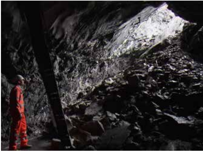
Fig. 2: Collapsed tunnel
