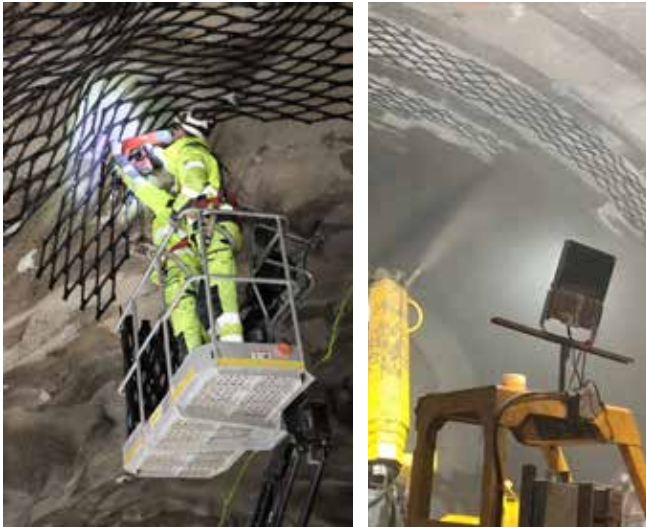
Fig. 5: Installing Dolenco Drain to tunnel crown and next covering with another layer of shotcrete.
