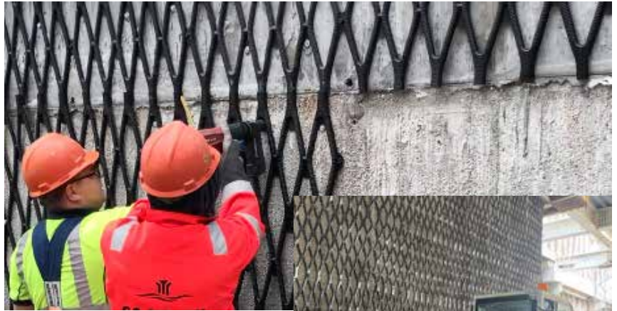
Fig. 8 (LEFT): Allowing shotcrete placement with water inflow using Dolenco Drain directly on the rock surface, with anchored wire mesh. Toronto, Canada
