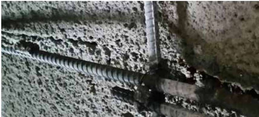
Steel Silo Lining Project
