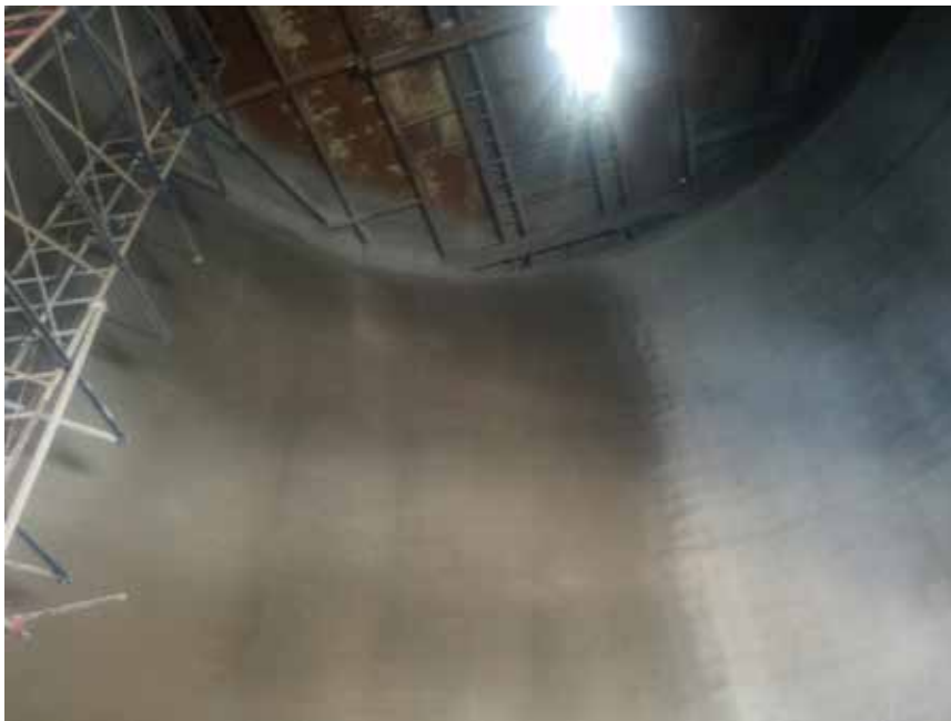
Steel Silo Lining Project
