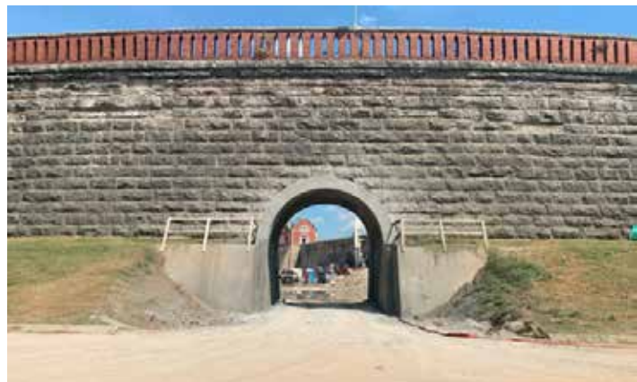
Nashville Tunnel Final
