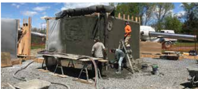
The concrete is in — almost finished cutting.
