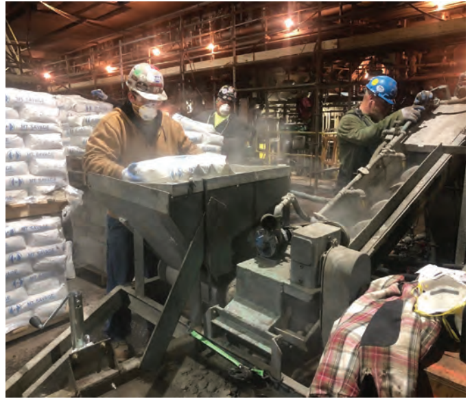
Fig. 5: Workers feeding prepackaged refractory
