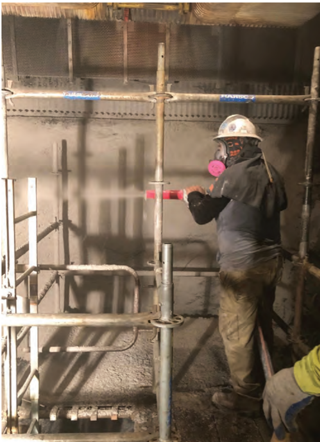
Fig. 1: Shotcreter placing refractory
