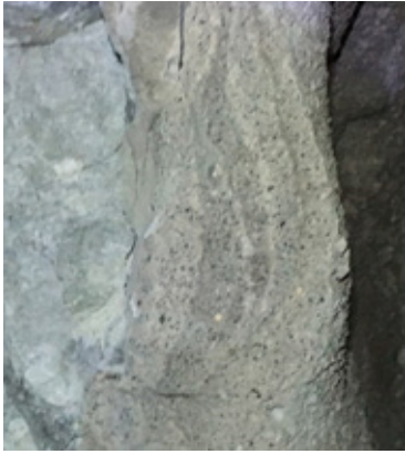
Fig. 4. Good bonding between shotcrete layers
