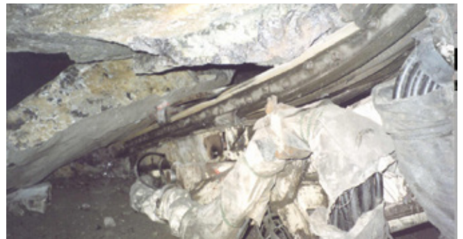
Fig. 1. Rock fall on jumbo equipment
