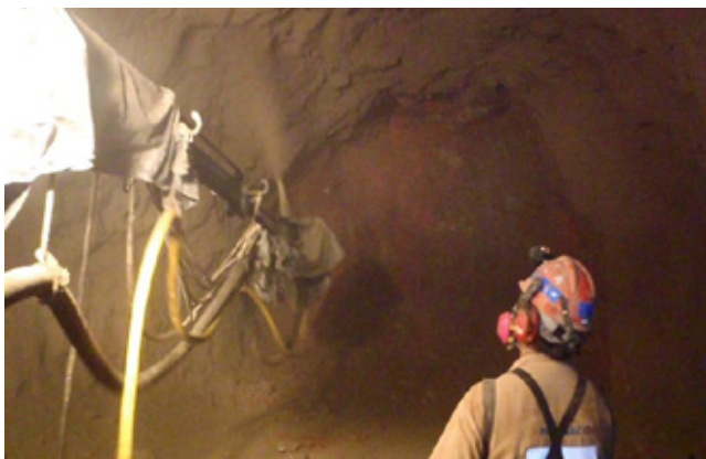
Fig. 2. Shotcrete placement with a remotely operated nozzle
