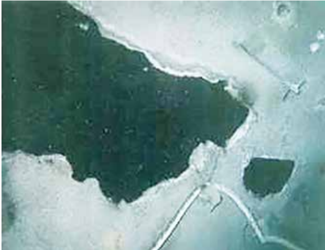
Fig. 2: Very-thin shotcrete
