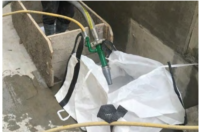
Fig. 5: Green Line G783-200 Fabric Concrete Placement Hose connected to a nozzle assembly utilizing a unique pipe.
