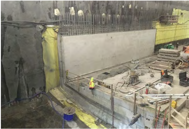
Fig. 22: Mount Pleasant Station, Box 4, South wall, invert slab level, 1.3 m thick.
