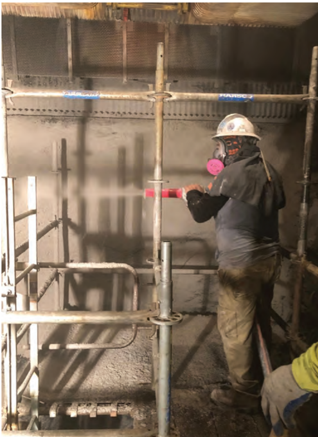
Fig. 1: Shotcreter placing refractory
