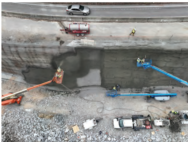
Fig. 3: Progress Photo of Geological Facing Installation and Sculpting.
