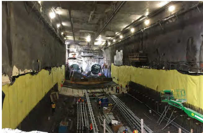
Fig. 2b: Sheet waterproofing membrane installation and invert slab construction.
