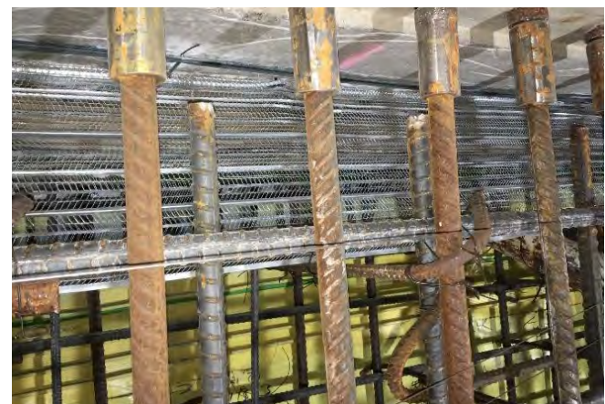
Fig. 10a: A 300 mm (12 in.) wide StayForm positioned 450 mm (18 in.) from front inner wall face.
