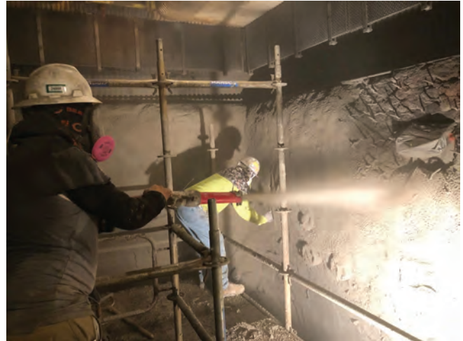
Fig. 2: Shotcreter in the foreground
