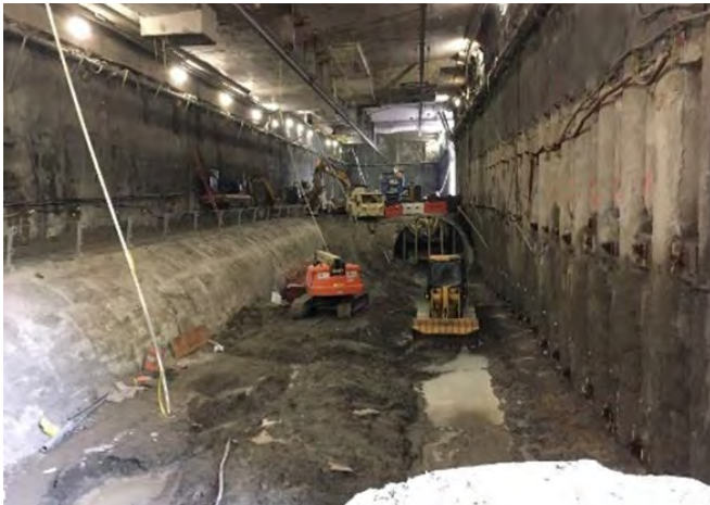
Fig. 2a: Top-down excavation and dismantling of precast tunnel segments.
