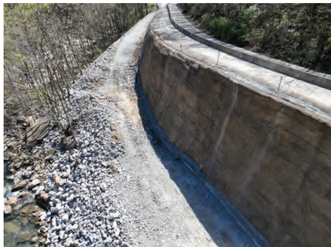
Fig. 4: Final Wall with Geological Facing, Facing South.
