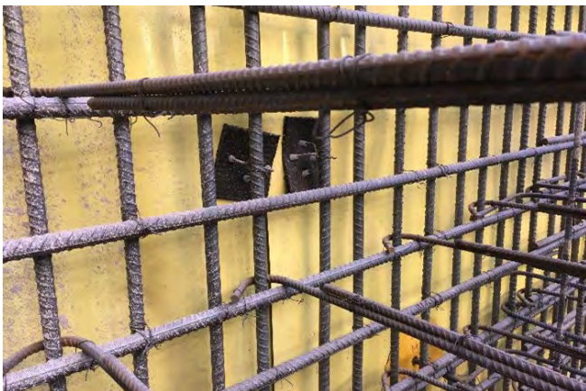
Fig. 14: Metal chairs to ensure cover is achieved. The chairs are specifically designed for shotcrete, enabling complete "wrap" of the chair with shotcrete.
