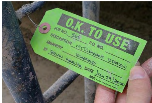
Fig. 8: Scaffold sign off indicating safe to use. Credit: Robert Mattes.
