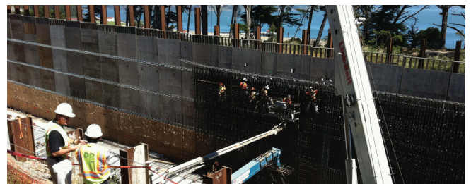
Blind Side Waterproofing
