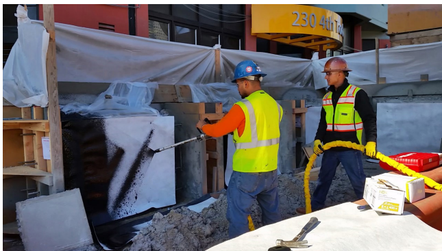
Fig. 3 Spray application of GTS gel on fleece reinforced HDPE
