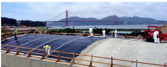
Positive Side Waterproofing
