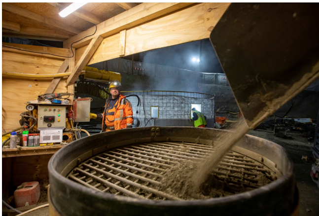
Fig.2: Feeding the Alivia-Pump with shotcrete
