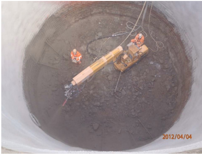
Fig.4: Normet spraying manipulator in action
