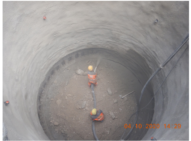
Fig.3: Shotcrete application inside the shaft
