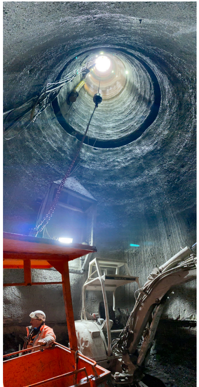
Fig.1: ventilation shaft from the excavation pit
