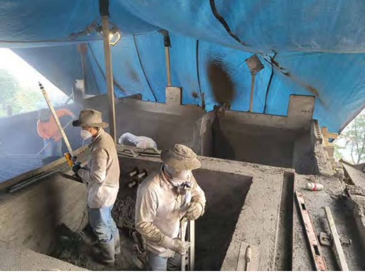
Fig. 6: Finishers working in spa under rain and shade tarp. Upside down boots keep tarp from punching through
