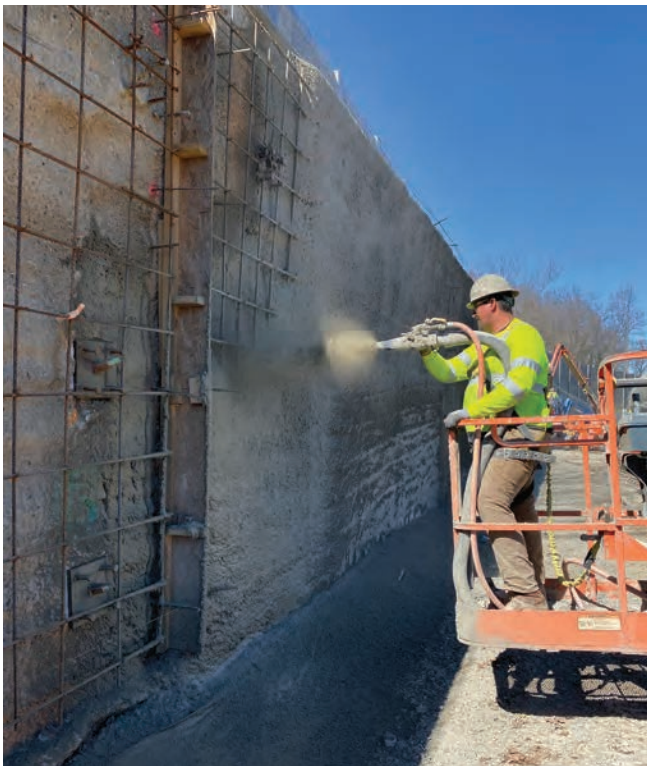
Shotcrete nozzlemen worked primarily from manlifts, shooting up to 70 cubic yards of material in a single day
