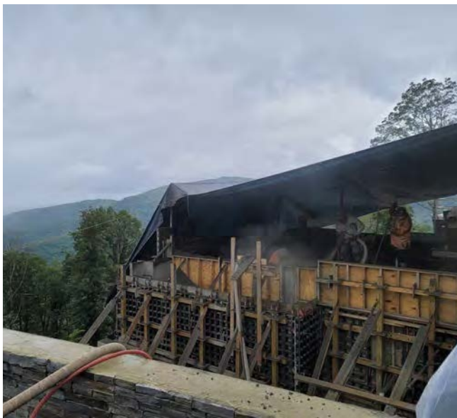
Fig. 3: Rain protection with a tarp. Nozzle man with an air lance operator at his side, keeping the adjacent material clean. Complex forming
