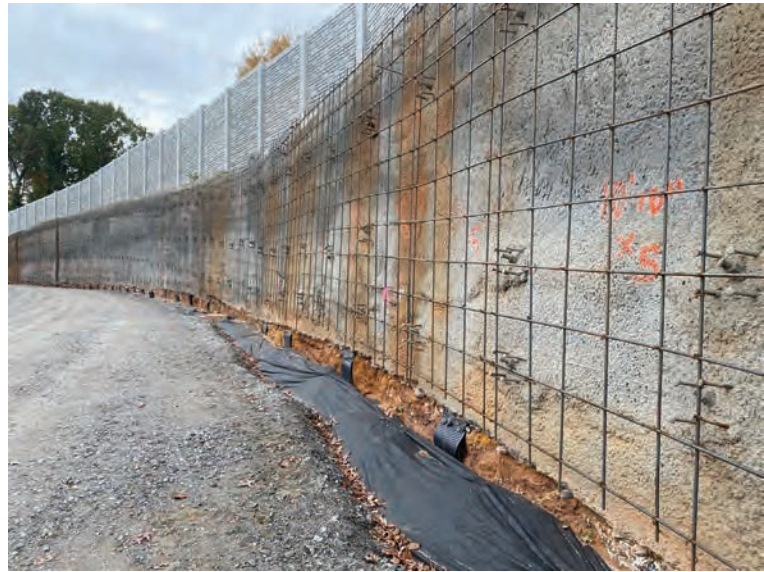
Once the soil nail wall was constructed, several layers of shotcrete were placed in front of it prior to carving the ashlar finish into the final two-inch layer
