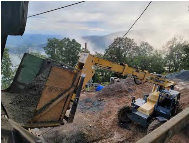
Fig. 7: Rebound removal
