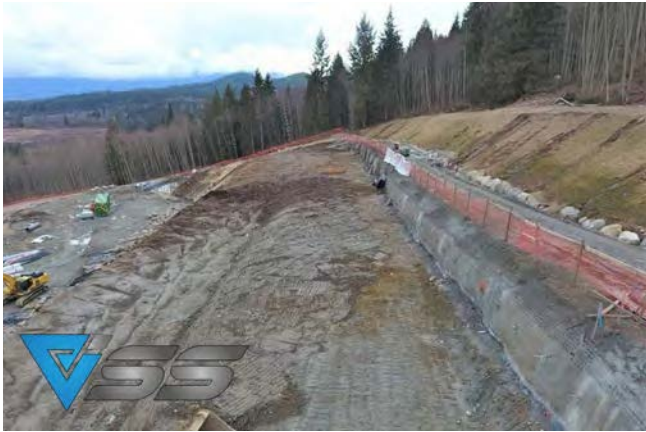
Fig. 2: Beginning of project
