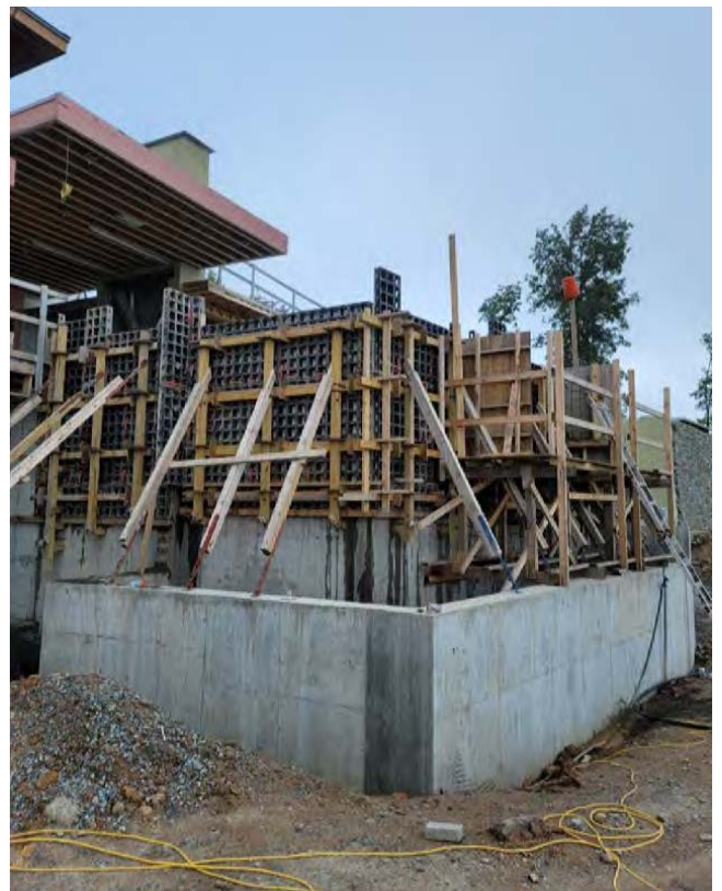
Fig. 5: Pour in place catch basin and foundation walls with forming above for shotcrete placed walls and catch basin floor
