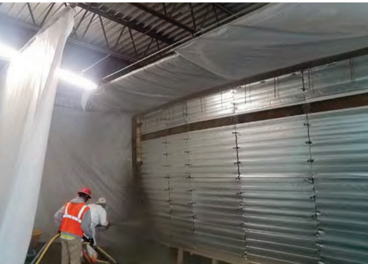
Fig. 6: shotcrete mockup warehouse
