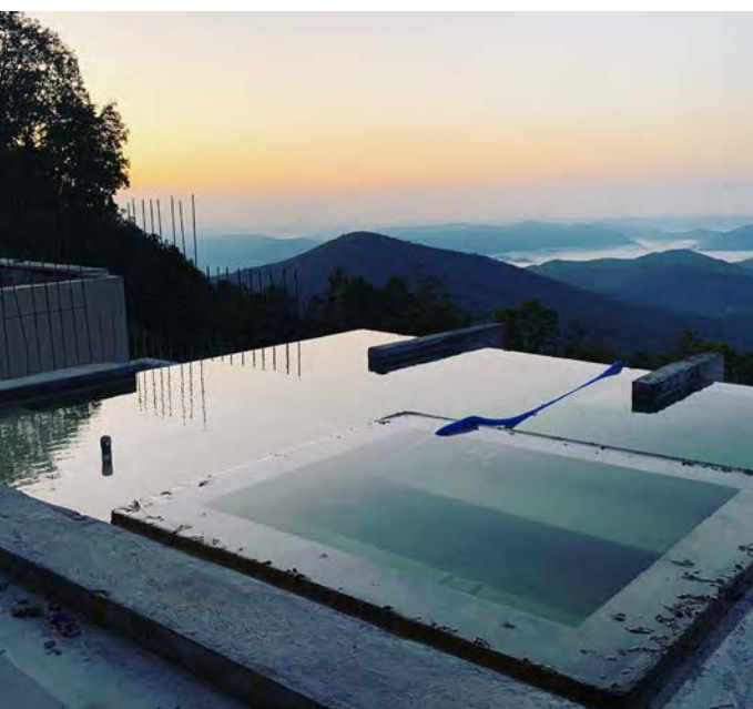
Fig. 12: Water Curing shell by flooding the project
