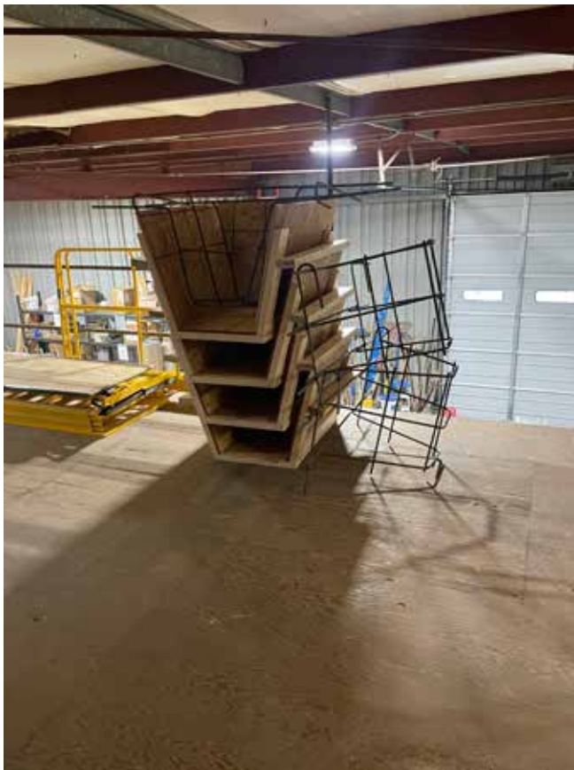
Fig. 2: Pre-formed skimmer boxes and rebar cages
