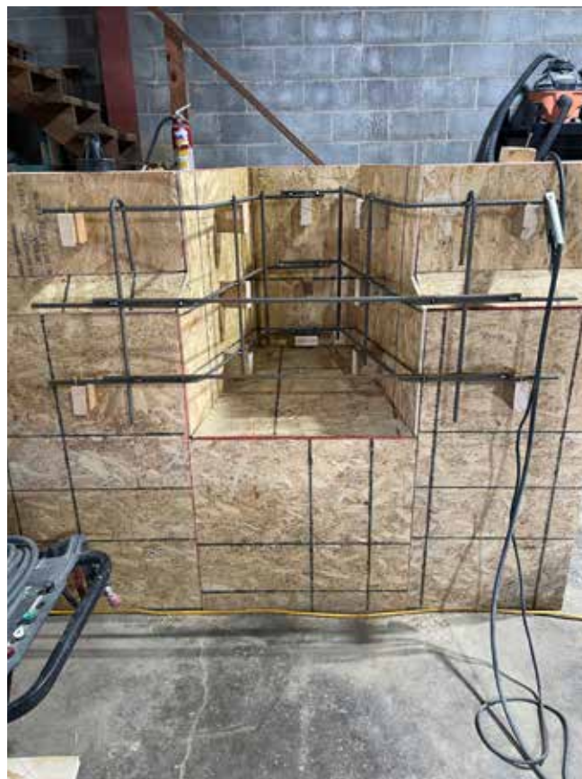
Fig. 3: Steel jig in place in mockup
