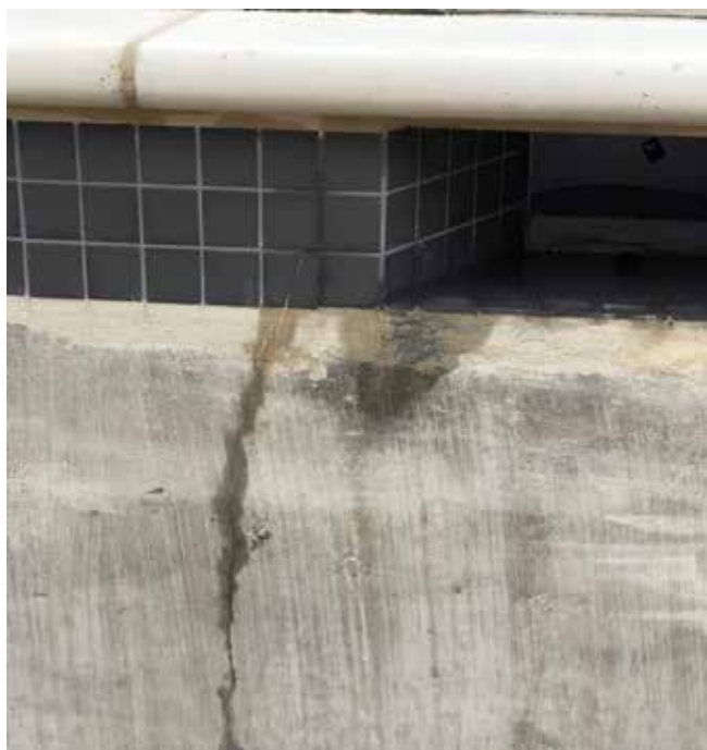
Fig. 7: Shrinkage crack at skimmer throat.
