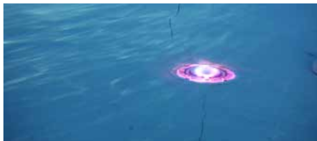
Fig. 8: Shrinkage crack at underwater light.
