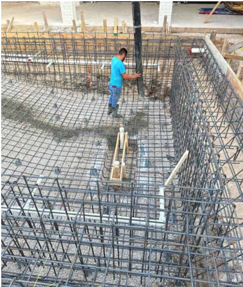
Fig. 2: Concrete placement in the floor of a pool with a boom pump.
