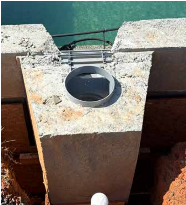
Fig. 5: After shotcrete placement during 28-day water cure.
