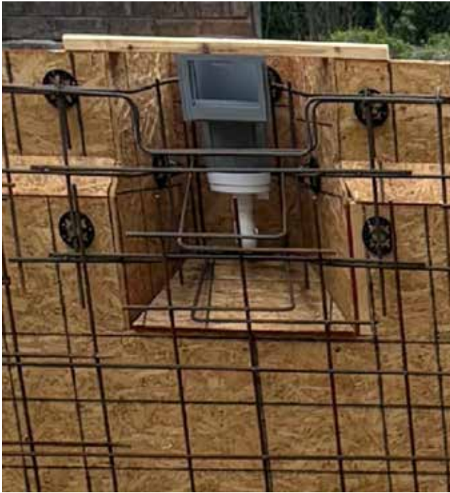
Fig. 4: Ready for shotcrete placement with reinforcement bars under the skimmer mouth and extra reinforcing steel in the box to control shrinkage.
