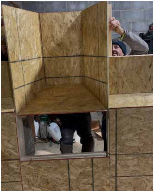
Fig. 1: Prefab box being installed on our mock-up wall
