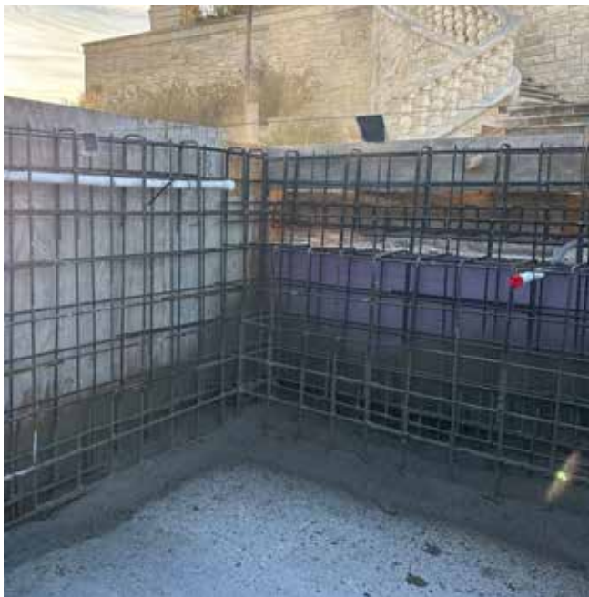
Fig. 4: Layer of shotcrete in place over the cast floor.
