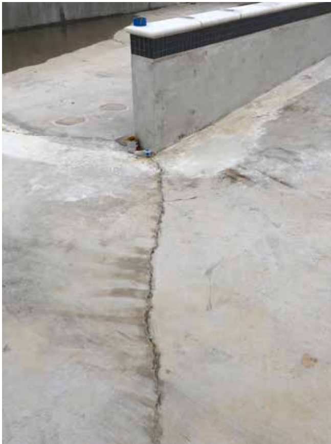
Fig. 5: Shrinkage cracks at reentrant corner.
