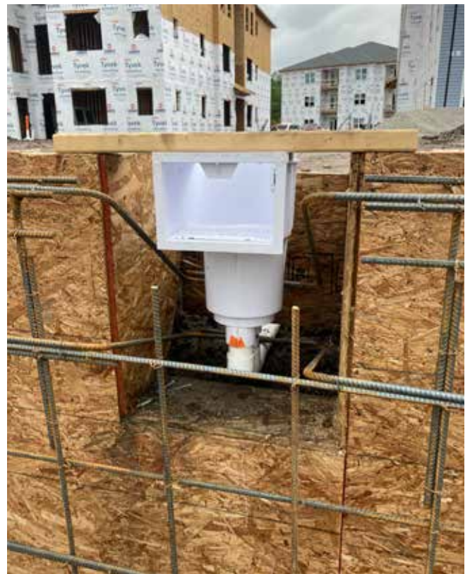
A typical skimmer box, rebar placement too close, forming too tight, not enough rebar across the skimmer mouth to continue the bond beam continuity.
