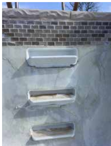
Fig. 8: Shrinkage crack at underwater light.
