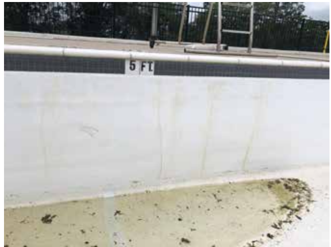
Fig. 5: Shrinkage cracks at reentrant corner.
