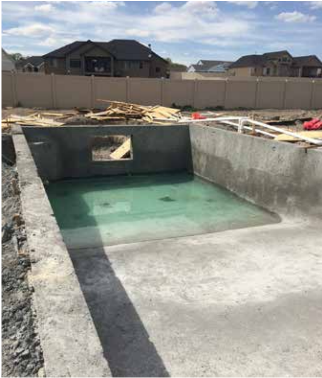
Fig. 3: Pool with ground water — hydrostatic relief valves in floor relieving hydrostatic pressure and allowing ground water to come up into shell.
