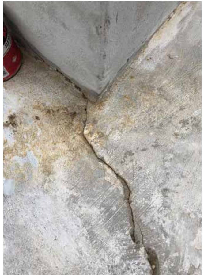
Fig. 2: Shrinkage crack worsened by freeze-thaw cycling.
