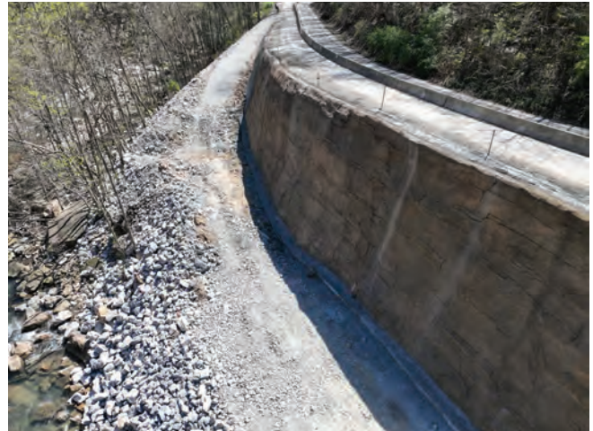
Fig. 4: Final Wall with Geological Facing, Facing South.
