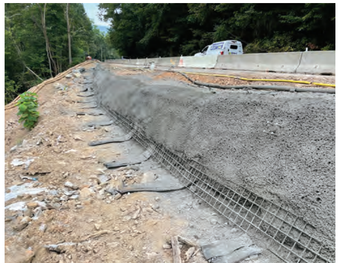
Fig. 2: Beginning Stabilization of SR 27.
