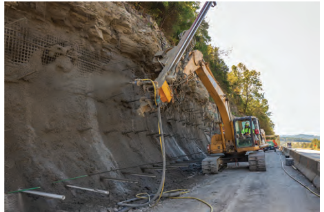
Fig. 1: Shotcrete Robot.
