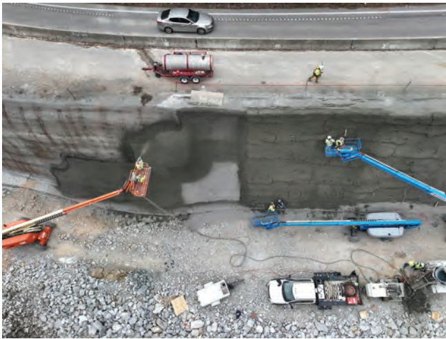
Fig. 3: Progress Photo of Geological Facing Installation and Sculpting.
