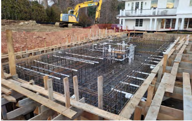
Fig. 3: Rigid forming, plumbing, and reinforcing steel installation.
