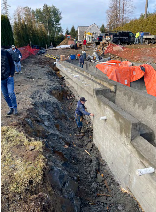
Fig. 4: Form removal—quality concrete example of the sprayed pneumatic wet shotcrete process.
