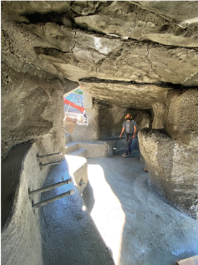
Fig. 2. Grotto roof and suspended slab finish.
